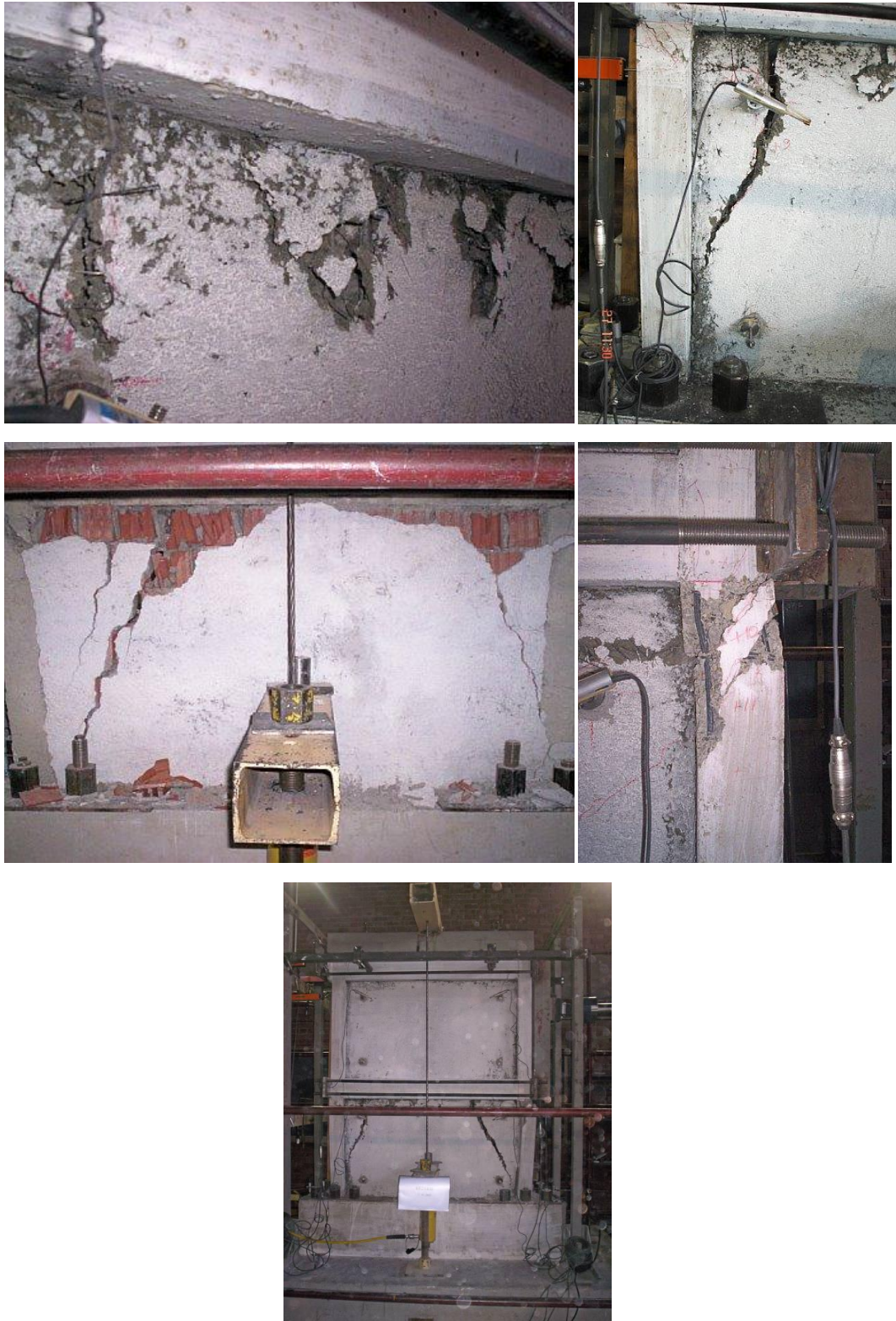
Figure 4.78 Views of TS10 (HF2ABM) Specimen during the Test
