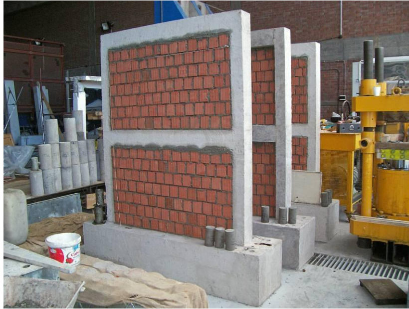
Figure 3.13 View of Brick Laying Application
