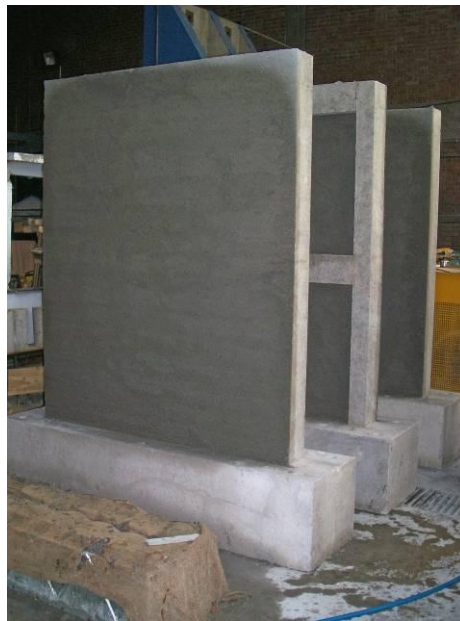
Figure 3.14 View of Plastering Application
