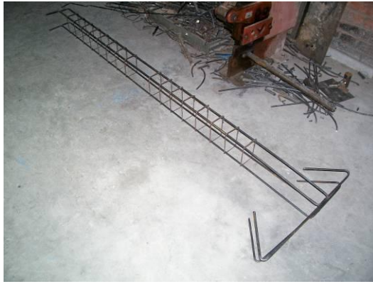
View of Column Reinforcement
