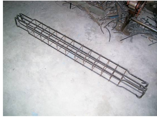
View of Beam Reinforcement
