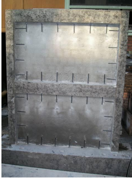
Figure 3.15 View of Anchoring Operation
