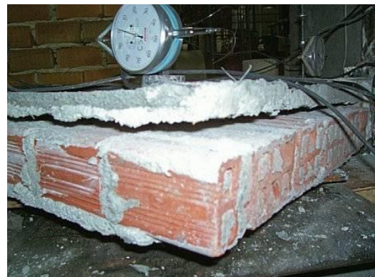
Figure 6.43 View of 2SSF1P-2
