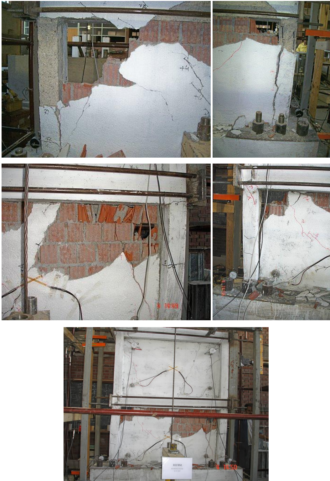
Figure 4.22 Views of TS1 (REFBM) Specimen during the Test
