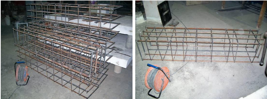
General View of Reinforcements View of Foundation Beam Reinforcement
