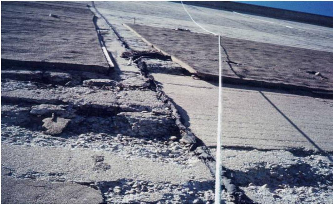
Figure 3.1 Deteriorated face slab of Salt Springs Dam (Scuero, 2007)
