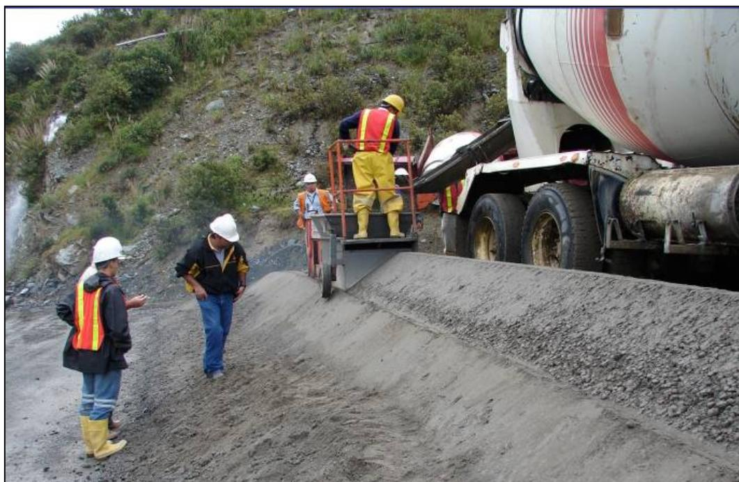
Figure 2.17 Site application of concrete curb casting (Orejuela, 2007)
