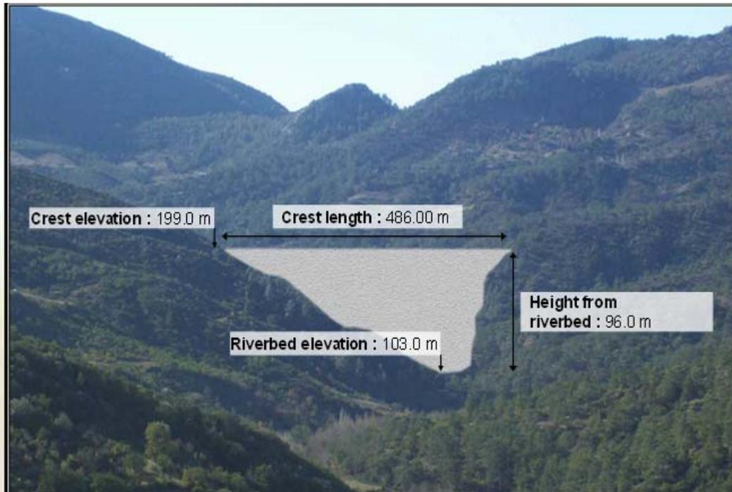
Figure 4.2 Proposed dam placement across Gökçeler River valley (Hidro Dizayn, 2007-b)
