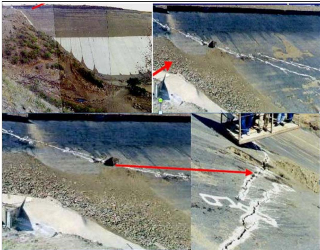
Figure 3.10 Cracking of face supporting zone at Xingó Dam (Souza, 2007)
