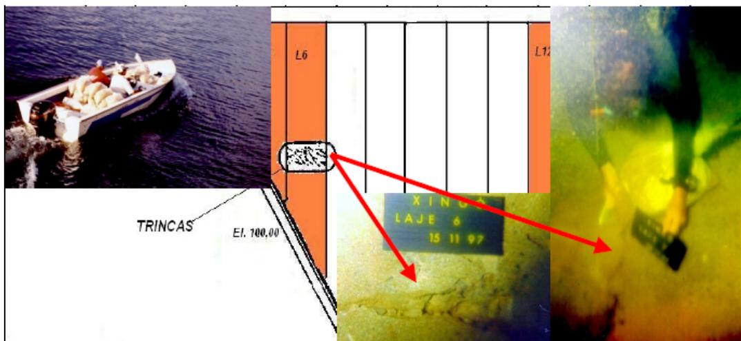
Figure 3.12 Underwater inspection of face cracks at Xingó Dam (Souza, 2007)
