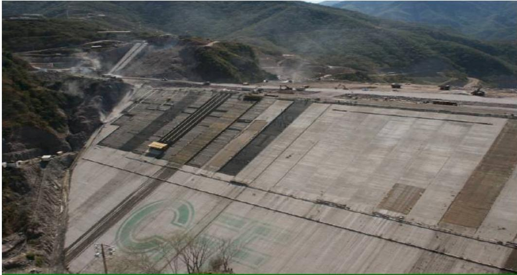
Figure 2.15 Site application of face slab construction (Marengo, 2007)
