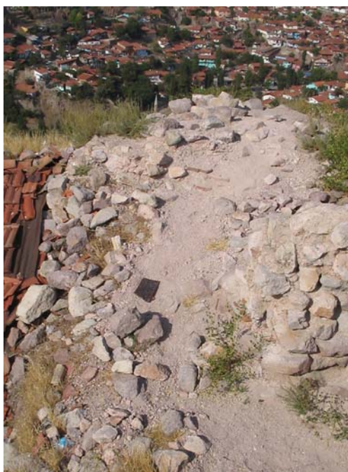
Figure 87. Rubble core, Bastion
