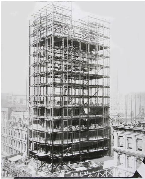
Figure 131. Reliance Building in Chicago under construction, August 1st 1894
