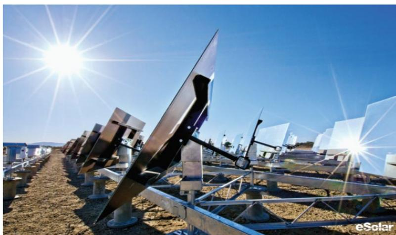
Figure 4.15 Heliostats developed by eSolar [124].
