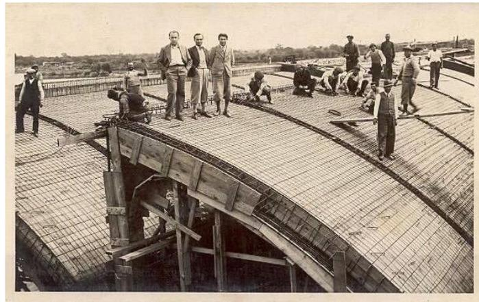
*Figure 3.14.* Construction of The Curved Roof And The Column (Source: <https://tr.pinterest.com/pin/427701295855019089/?lp=true>, accessed on 15.02.2019)
