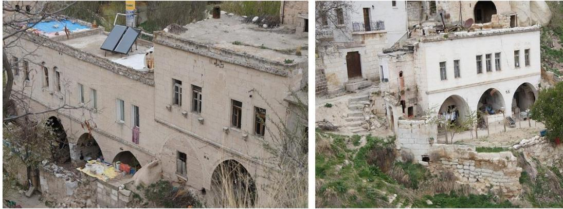
Figure 4.14. Buildings having their ground floor units arranged side by side (Type 1.G.a seen in Figure 4.18)
