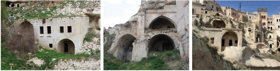
Figure 3.11. Examples of mixed technique, extending from rock-cut spaces with masonry units
