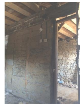
5. Room 1 - timber frame partition wall
