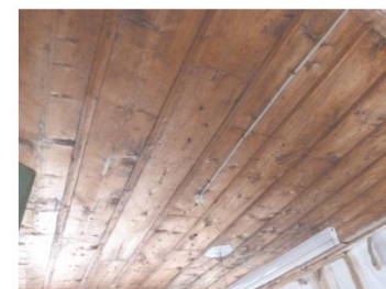
12. Room 3 - timber ceiling planks
