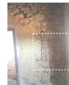
11. Hall - filled-in window opening
