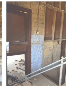
9. Hall - timber frame partition wall and timber door
