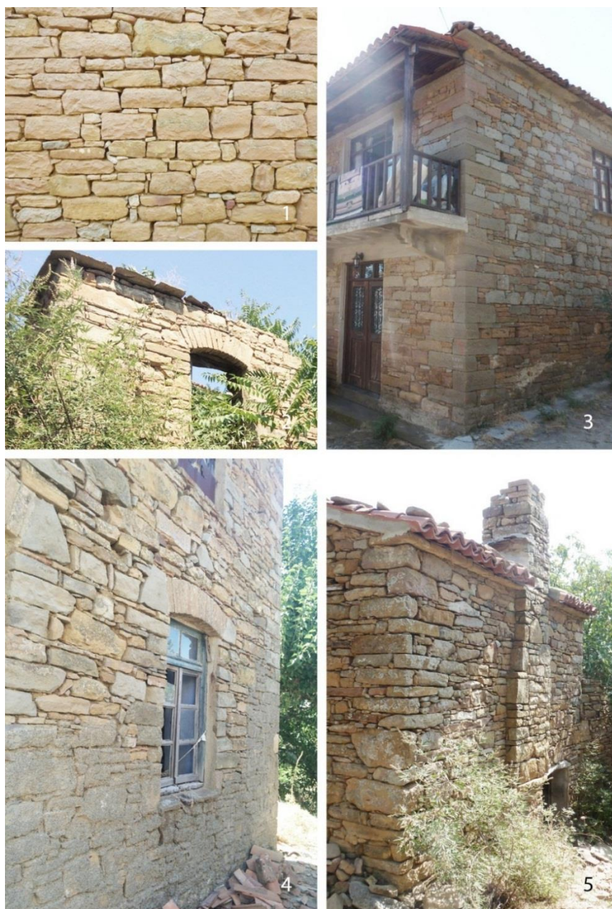
Figure 94: Zeytinliköy, stone masonry details: (1) masonry technique; (2) wall and window end details; (3) cornerstones; (4) stone masonry and window opening; (5) chimney detail – kremasti
