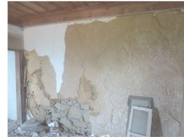
10. Room 2 - mud mortar on the stone wall
