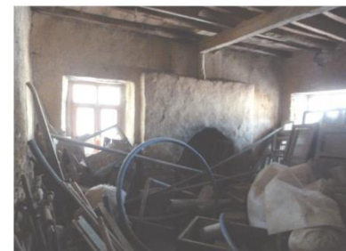
6. Room 1 - mud mortar wall finishing material
