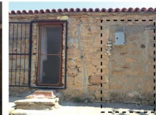
4. Filled-in door opening in the west facade
