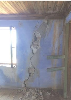
11. Room 2 - structural crack
