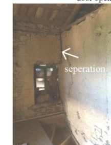
9. Hall- intersection of the partition wall and south wall
