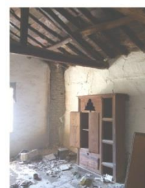
12. Hall -timber roof system
