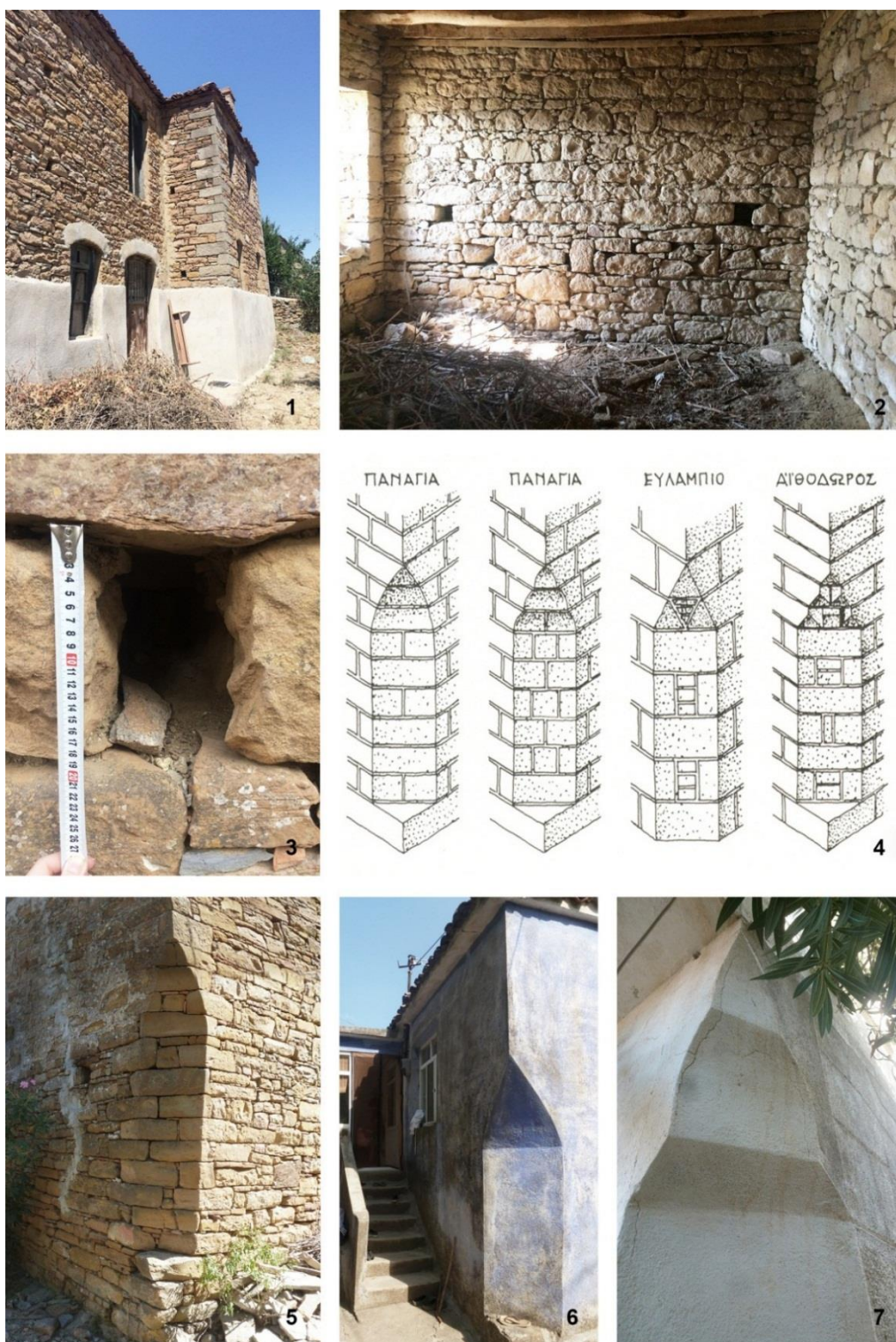
Figure 96: Zeytinliköy, stone masonry details: (1) ventilation holes on a facade; (2) view of ventilation holes from the inside; (3) dimensions of a ventilation hole; (4) drawings of regularly cut corner stones (Pasadeos 1973, appendices ΠΙΝ:9); (5-7) examples of corner stones
