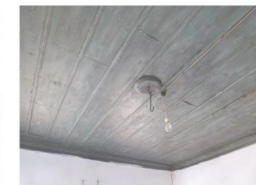
14. Room 5 - timber ceiling planks oil painted
