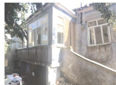
2. Reinforced concrete addition in the entrance
