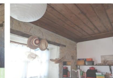
13. Room 4 - timber lintel and ceiling
