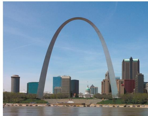
Gateway Arch, Eero Saarinen Catenary arch, 192m in height and the length
