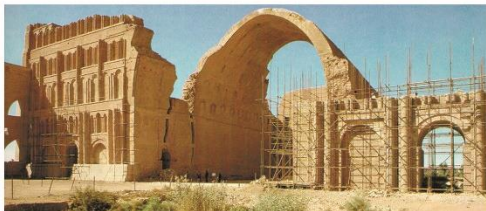
Catenary arch structure of Taq Kasra. AD. 540
