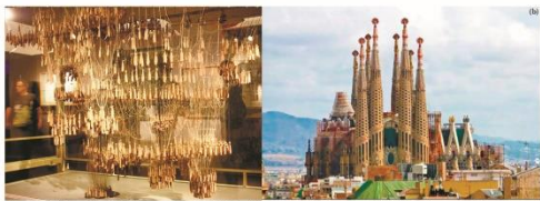
Figure 10 (a) Chain model and (b) the constructed cathedral of Gaudi's Sagrada Familia (Source photo 10 (b) Wikipedia commons file)
