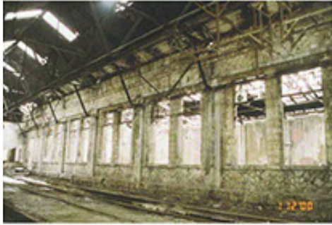
Figure 95 The exterior wall of the Atelier 3 which is the interior wall of the hangar building before the restoration. (Source: https://www.cermodern.org/hakkimizda.html )
