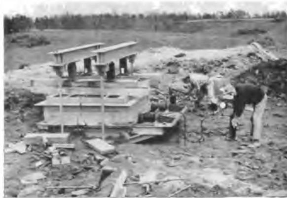
*Figure 2.8. Arrangement of an In-Situ Large Scale Direct Shear Test (Sowers et al., 1961)*
