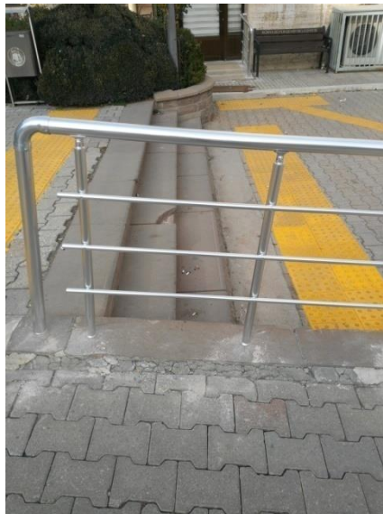
Figure 4.43. Stairs with tactile surface and handrail
