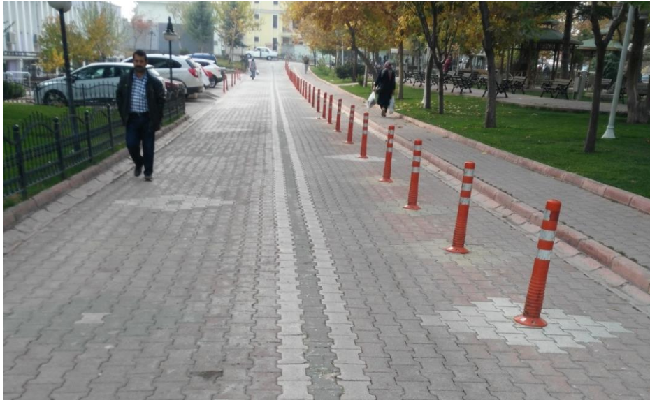
Figure 4.26. Pavement with no changes in level
