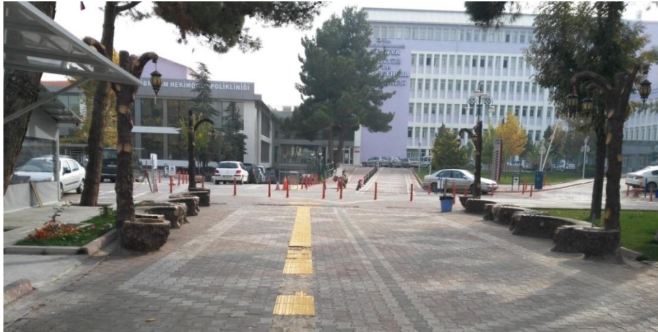
Figure 4.21. Discontinuous and interrupted walking surfaces
