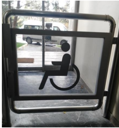
Figure 4.52. Entrance for wheelchair users
