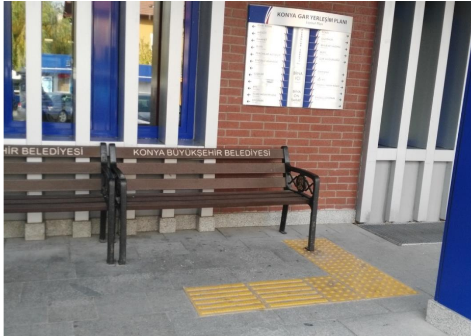
Figure 4.7. A discontinuous and non-functional tactile walking surface
