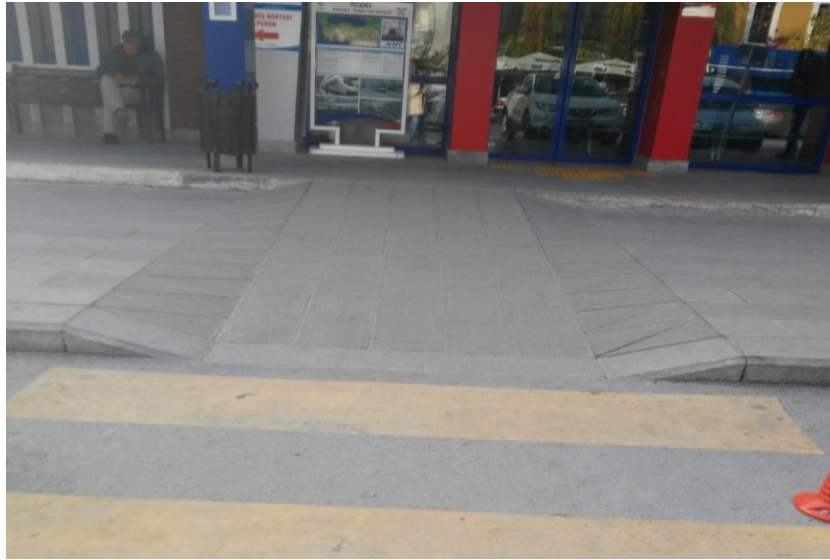
Figure 4.4. A curb ramp intersecting pedestrian crosswalk
