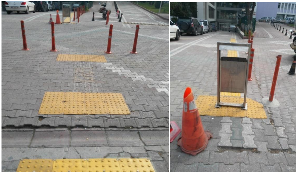
Figure 4.22. Tactile surfaces occupied by different materials
