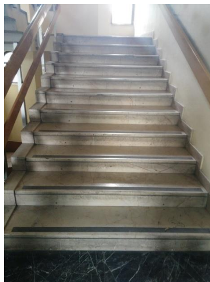
Figure 4.55. Stairs with handrails at both sides and slip-resistant strip
