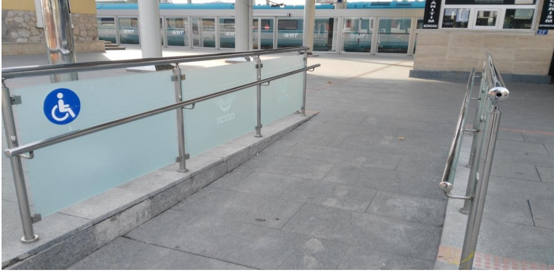
Figure 4.6. A ramp for wheelchair users
