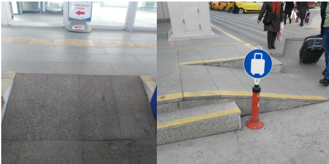
Figure 4.11. Vertical ramps not having tactile walking surfaces
