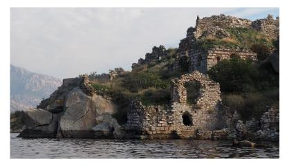
Figure 4.37: Küçük İkiz Ada Monastery, the deterioration of the remains due to the water level
