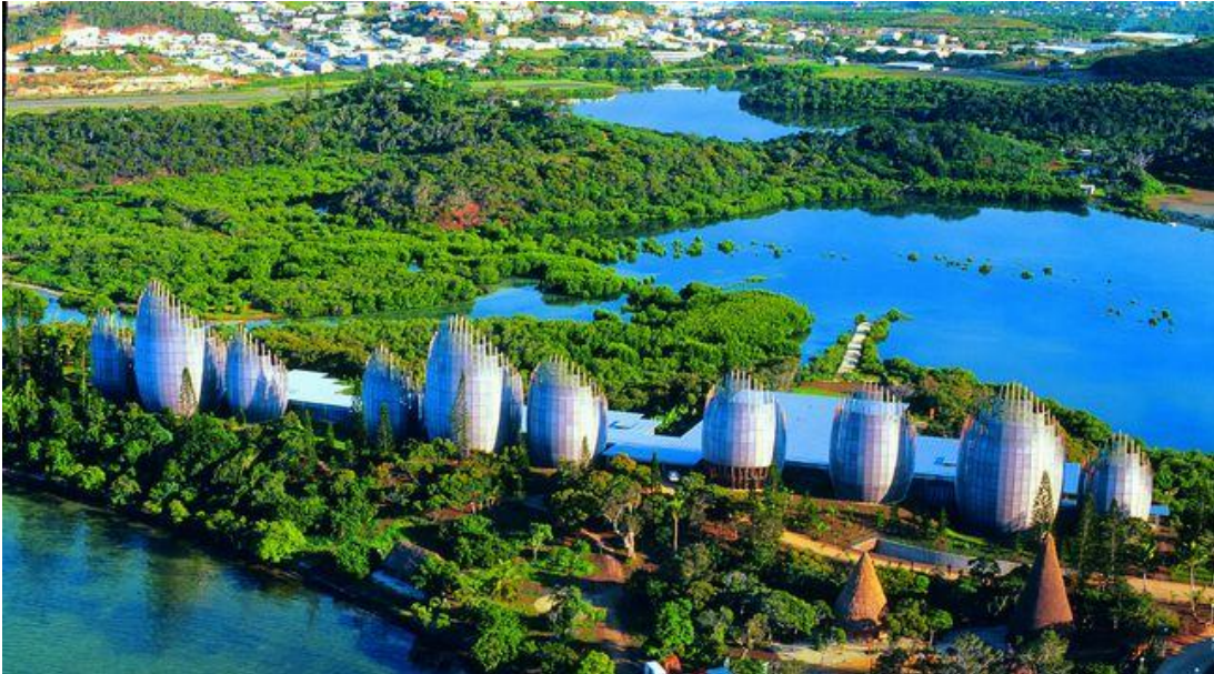
Figure 4.42 Aerial view of the Kanak Culture Center (Photograph: [Internet, WWW] Address: https://www.connaissancedesarts.com/archi-jardin-et-patrimoine/renzo-piano-au-diapason-1113634/ )
