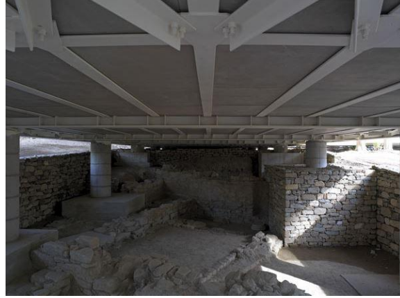
Figure 4.48 Archaeological remains under the museum and the steel structure of the building. (Photograph: [Internet, WWW] Address: http://www.arkiv.com.tr/proje/afrodisyas-ek-muzesi/1410 )
