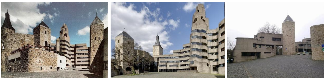
Figure 4.13 View of Old Bensberg Castle and Town Hall from entrance. (Figure: [Internet, WWW] Address: https://www.competitionline.com/upload/images/c/f/9/f/0/6/5/9/cf9f0659fe4cf6b7c98ea806ffd939e2_1.jpg )
