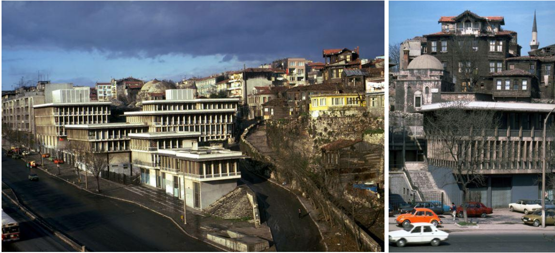
Figure 4.51 General view of the Zeyrek Social Security Building. (Photograph: [Internet, WWW] Address: http://www.arkiv.com.tr/proje/sosyal-sigortalar-kurumu-tesisleri-zeyrek/3226 )
