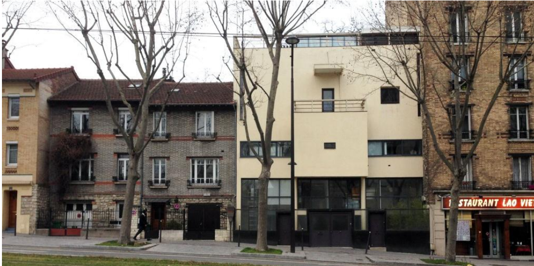
Figure 2.12 View of the Maison Planeix from boulevard. (Photograph: [Internet, WWW] Address: https://www.mimoa.eu/images/47013_1.jpg )
