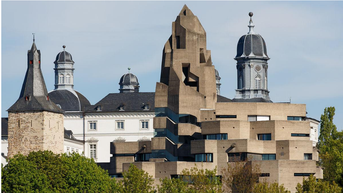
Figure 4.22 Town Hall's staircase tower in Bensberg skyline with other baroque and medieval towers. (Photograph: [Internet, WWW] Address: https://www.atlasobscura.com/places/bensberg-old-castle )
