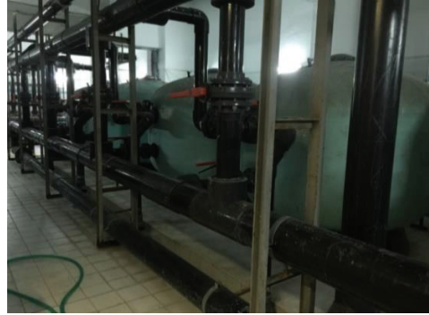
Figure 54. Chlorine Dosage and Acid Tanks (Left) and Sand Filters (Right).
