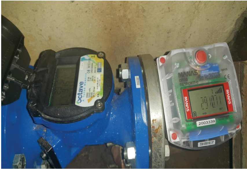
Figure 26. A Smart Water Meter installed in the METU Campus
