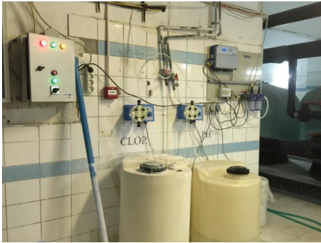
Figure 54. Chlorine Dosage and Acid Tanks (Left) and Sand Filters (Right).
