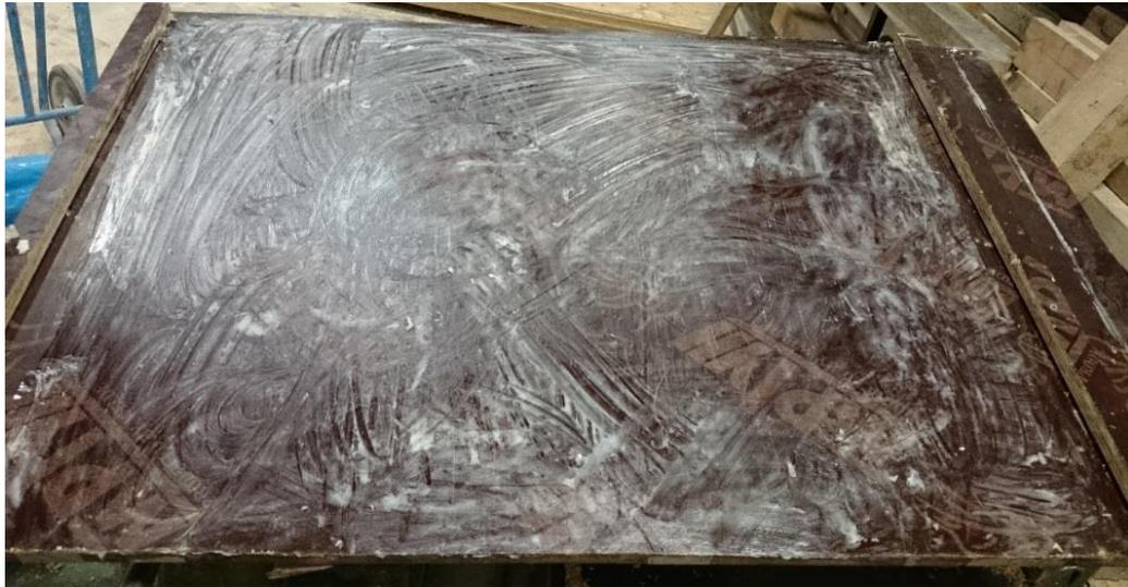
Figure 2.26 Vaseline on the formwork
