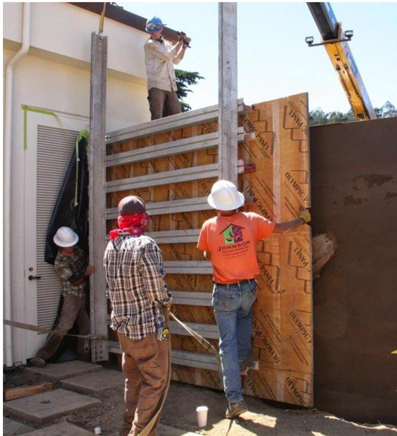
Figure 2.20 Bigger formwork system (URL – 8)
