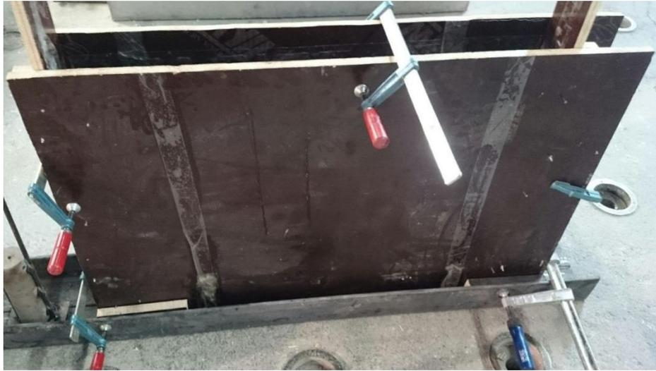
Figure 2.27 Preparation of formwork
