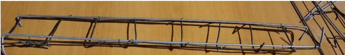
Figure 2.43 Horizontal reinforcement with tie bars
