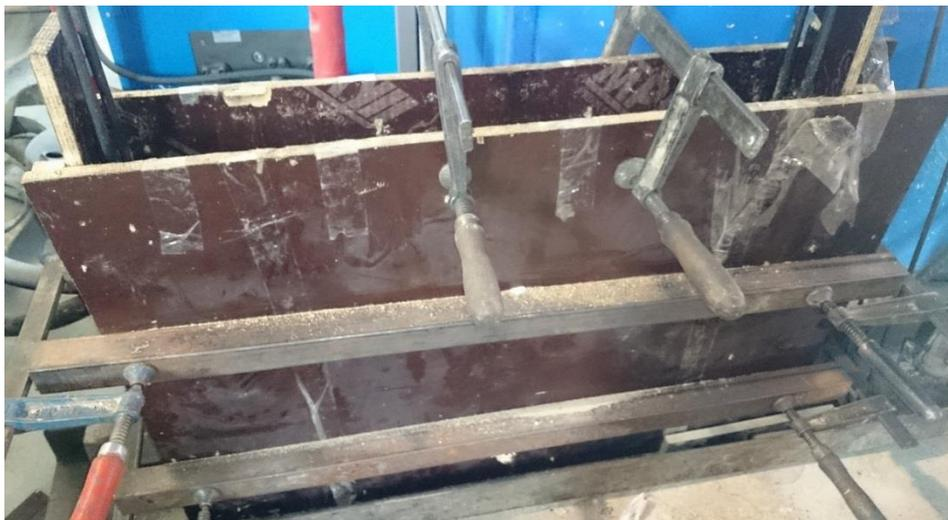
Figure 2.28 Formworks with supports
