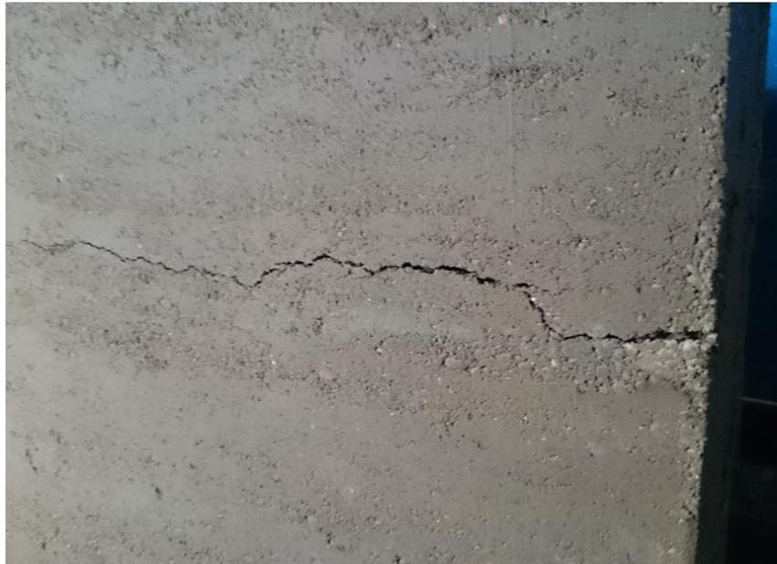
Figure 3.42 Cracks because of shrinkage
