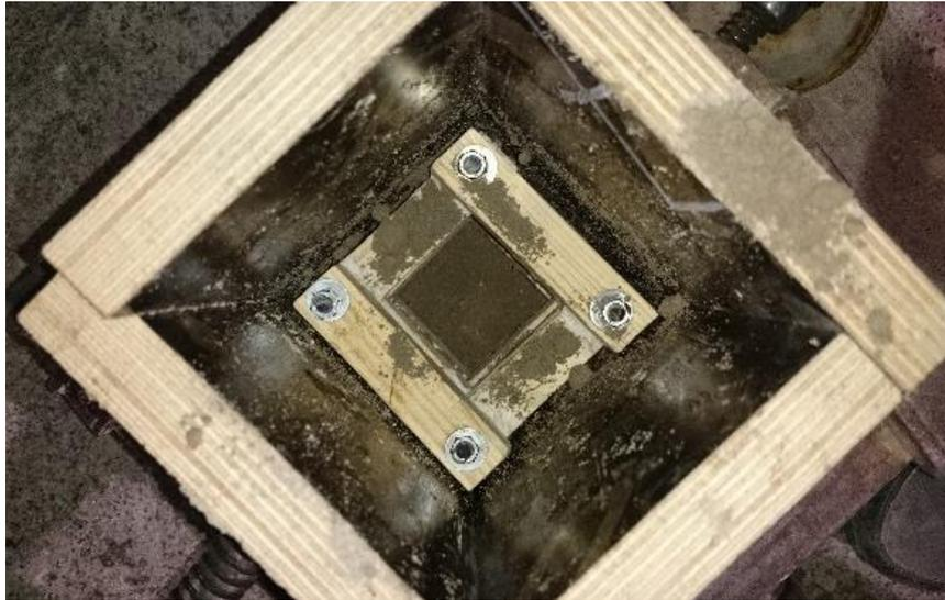
Figure 2.11 Formwork for wooden reinforced column
