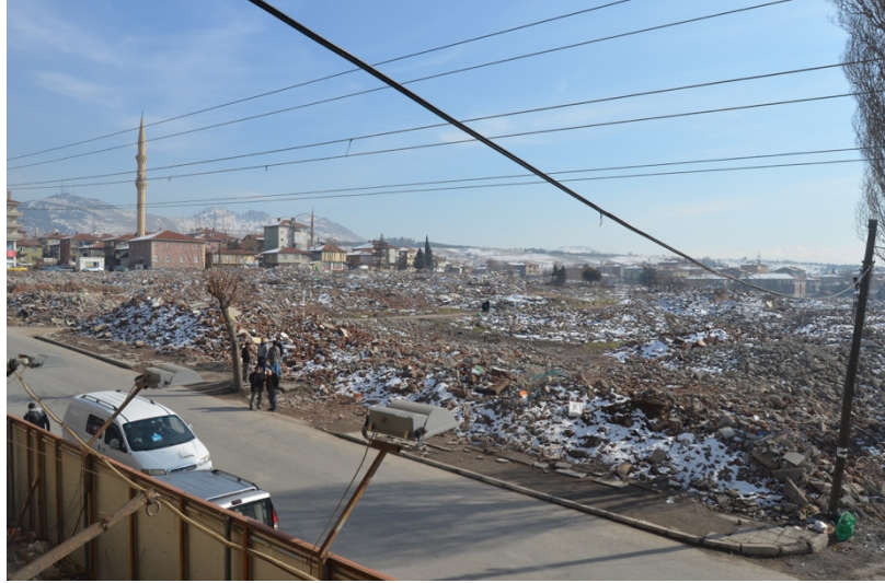
Figure 3.7 Önder neighborhood after demolishments for urban transformation (Source: Personal archive, 2016)
