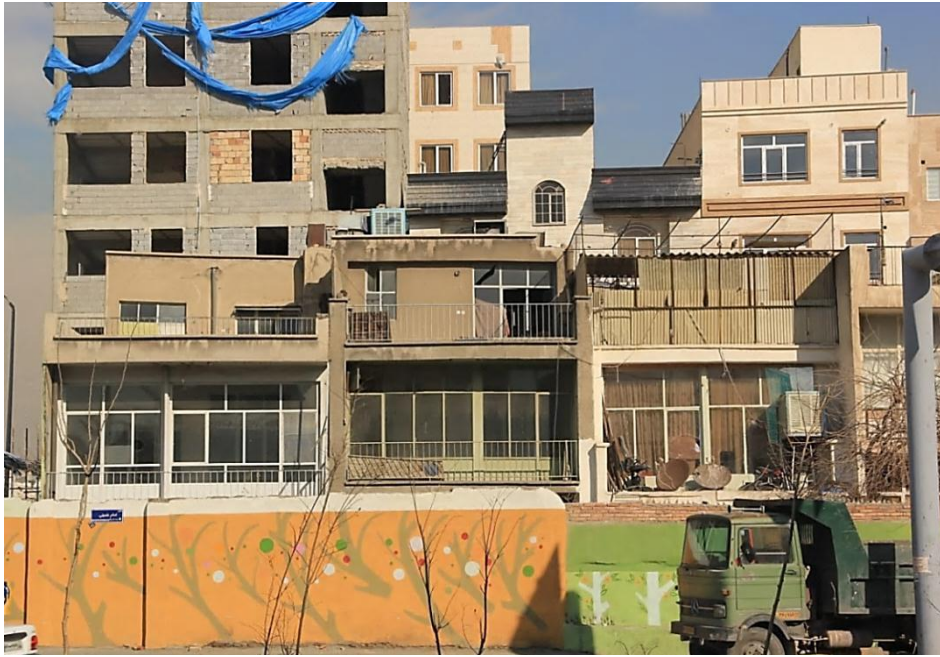
Figure 145: Covered Balconies. Balconies because of noise pollution and air pollution have been covered with plastic sheets, matting, fabric in Emam Khomeini district of Tehran. (Photo was taken by author, December 2015)
