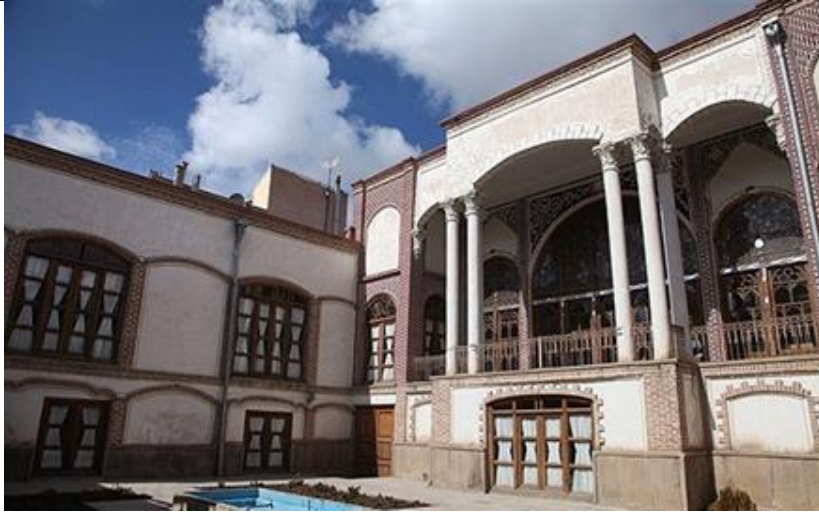
Figure 90: Heydarzade House. Tabriz, Cold Region of Iran
