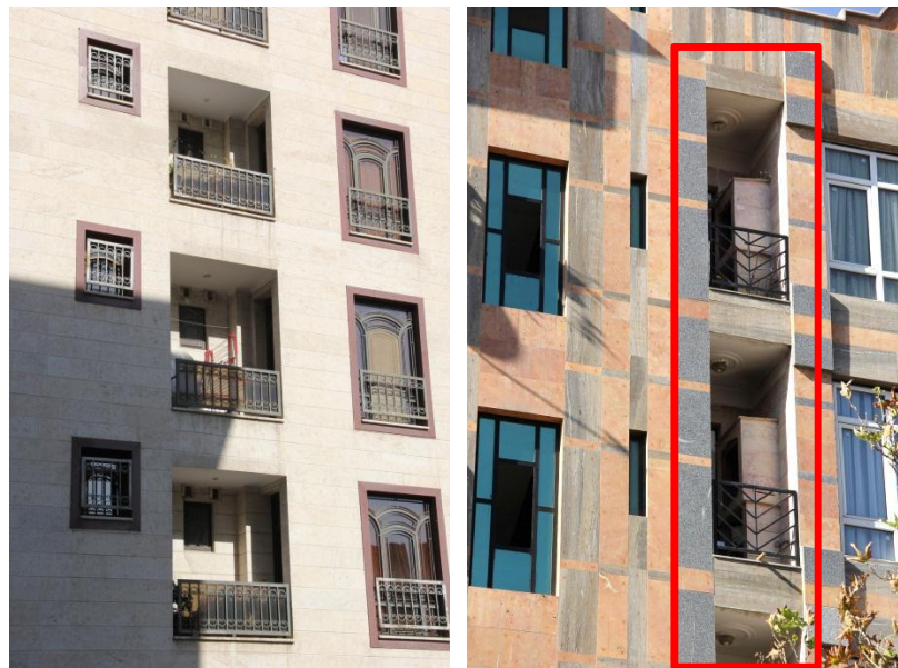
Figure 138 & 139: Small Balconies. Low area spaces make balconies useless spaces in residential buildings. Shahrak Gharb district of Tehran. (Photo was taken by the author, September 2016)
