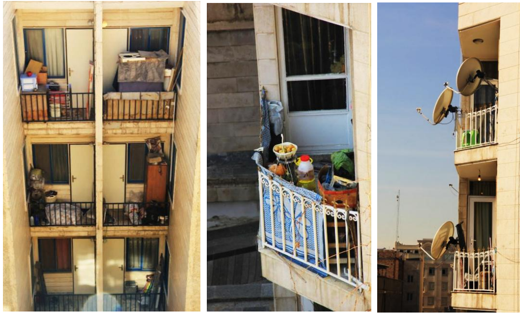
Figure 116, 117 & 118: Balconies as Warehouse. Saadat Abad district of Tehran
