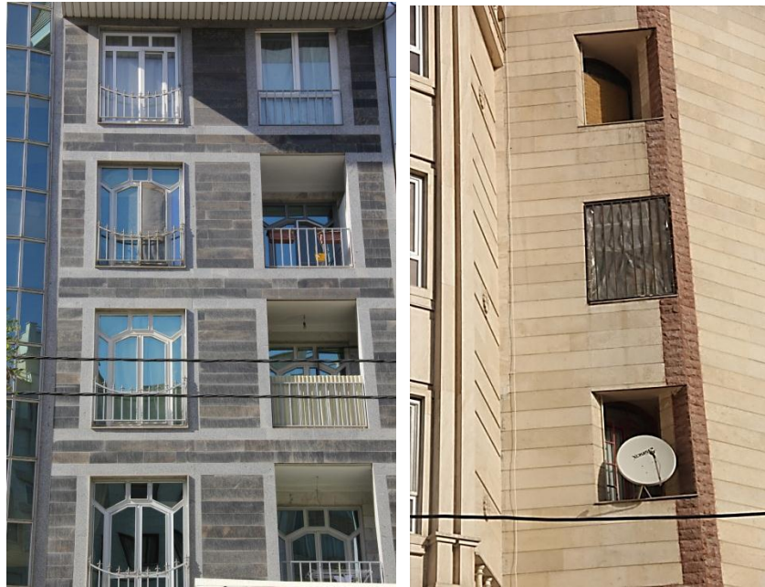
Figure 136 & 137: Small Balconies. Low area spaces make balconies useless spaces in residential buildings. Narmak district of Tehran. (Photo was taken by the author, December 2015)
