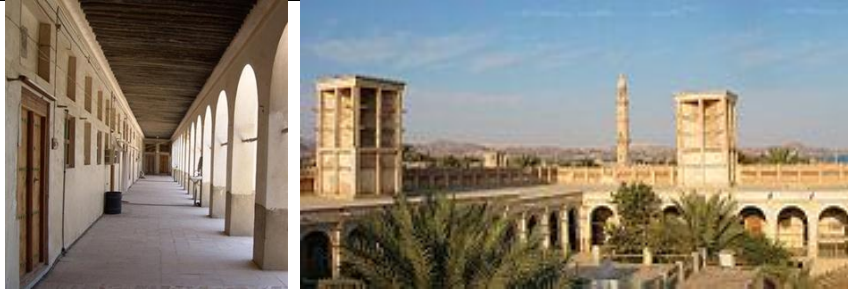
Figure 84 & 85: The Loggia (Ravagh in Persian)of Golbatan House. Hormozgan, the Southern Hot and Humid Region of Iran
