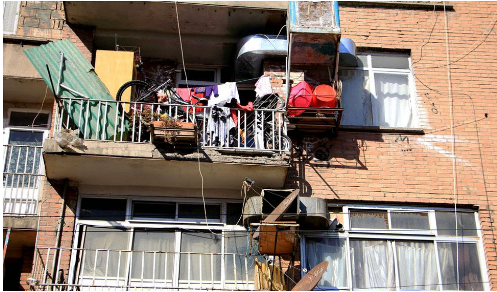
Figure 12: Misusing of Balconies in Tehran
