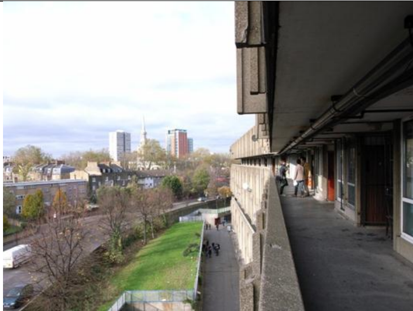
Figure 72: A Street in the Sky. Robin Hood Gardens building. Source: https://commons.wikimedia.org/wiki/File:Robin_Hood_Gardens_Streets_in_the_Sky.jpg (last retrieved on 10 may 2016, at 16:00)
