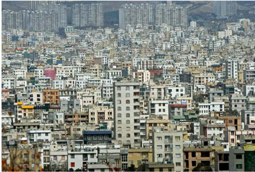
Figure 154: Visual Pollution Caused by Unpleasant Heterogeneous Constructions.
