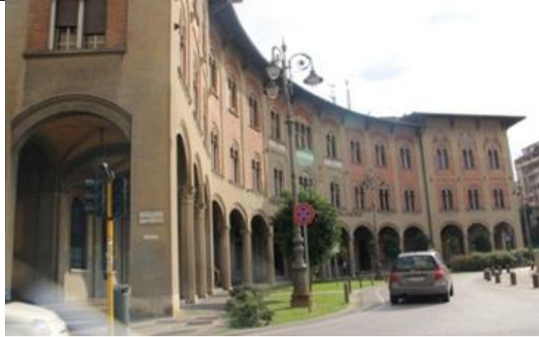
Figure 77: Loggia (Photo taken by author, 2016)
