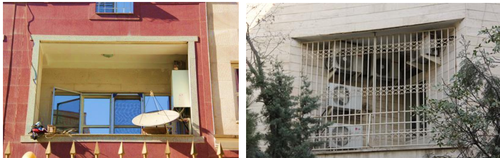
Figure 8 & 9: Misusing of Balconies in Tehran
