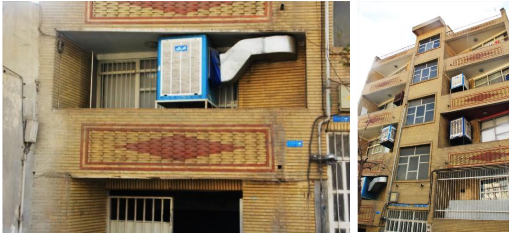
Figure 122 & 123: Balconies with Different Functions. Locating heating appliances and air conditioners in balconies
