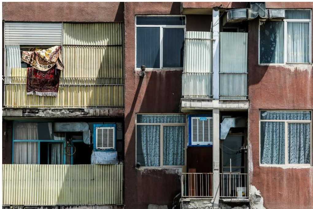
Figure 3: Misusing of Balconies in Tehran
