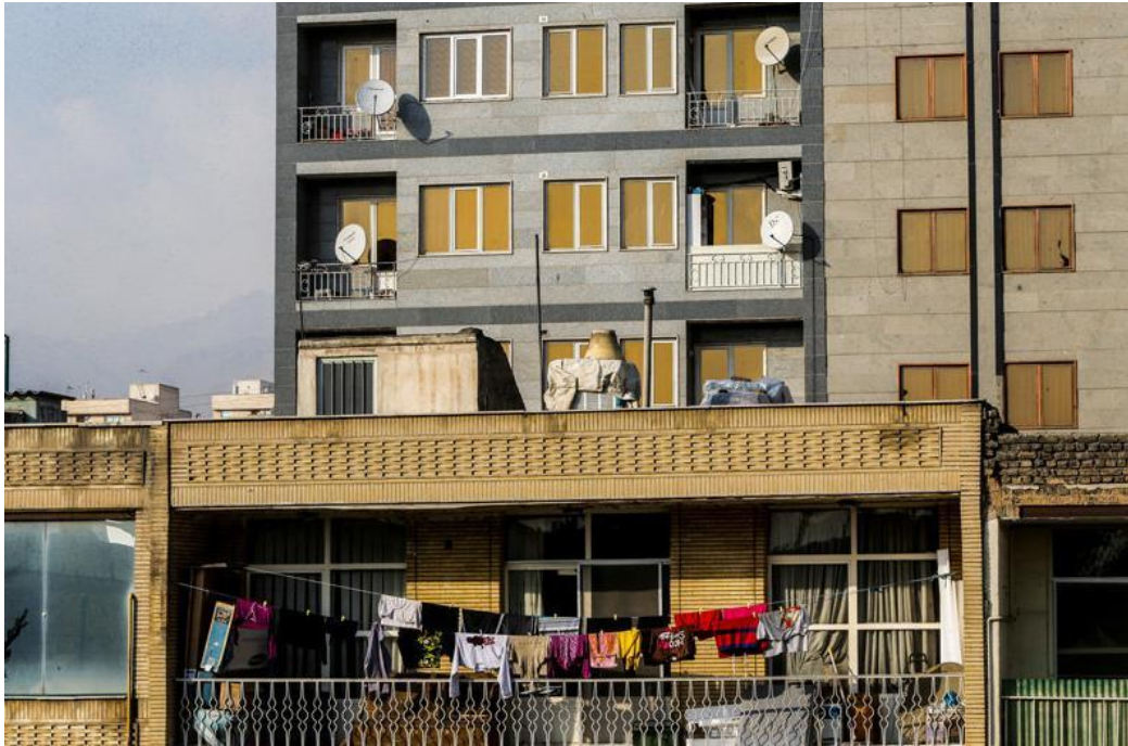
Figure 10: Misusing of Balconies in Tehran Source: http://www.peykeiran.com (Last retrieved on 16 September 2015, at 10:15)
