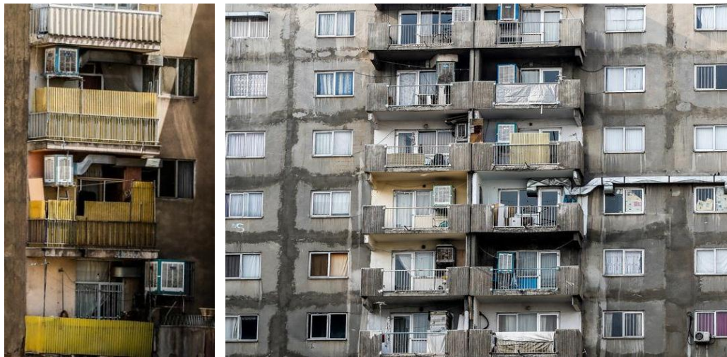
Figure 1 & 2: Misusing of Balconies in Tehran
