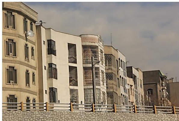
Figure 157 & 158: Visual Pollution Causing by Walls and Fencing. (Photo was taken by author, December 2015)
