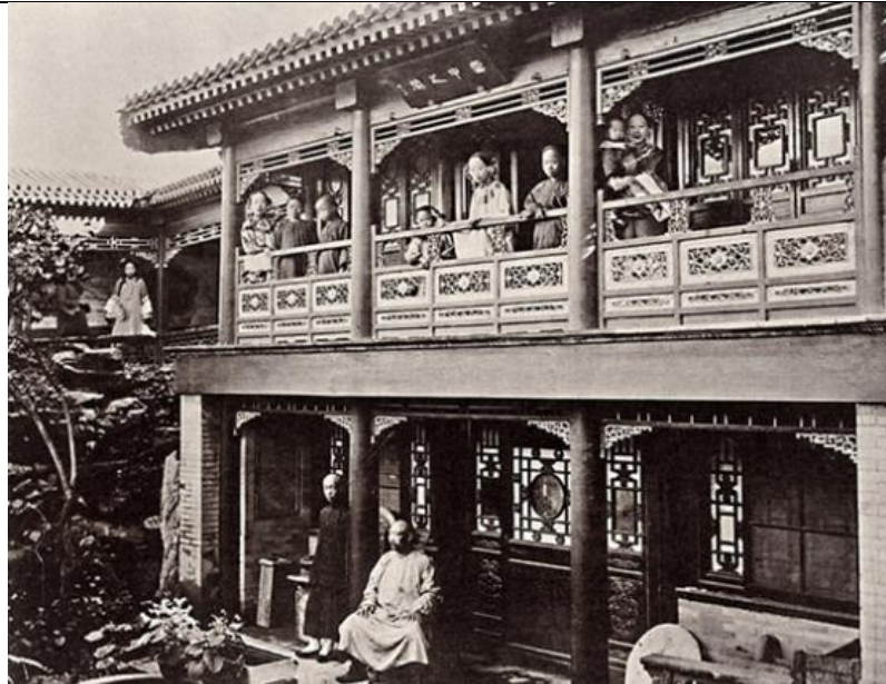
Figure 65: Xi Shi Railing
