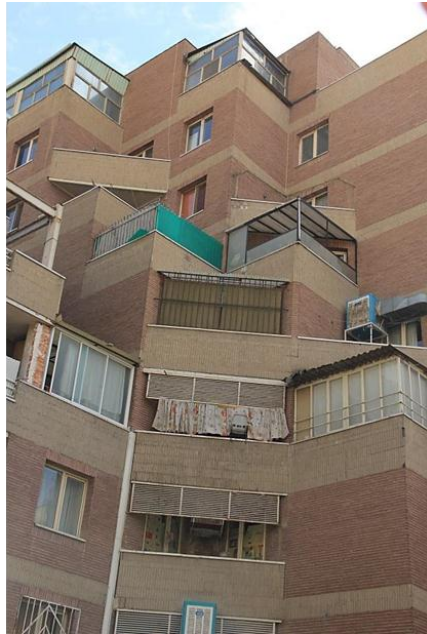
Figure 163: Untidy Balconies. Visual pollution caused by an unpleasant face of messy balconies in urban space of Tehran Navab district of Tehran. (Photo was taken by author, December 2015)
