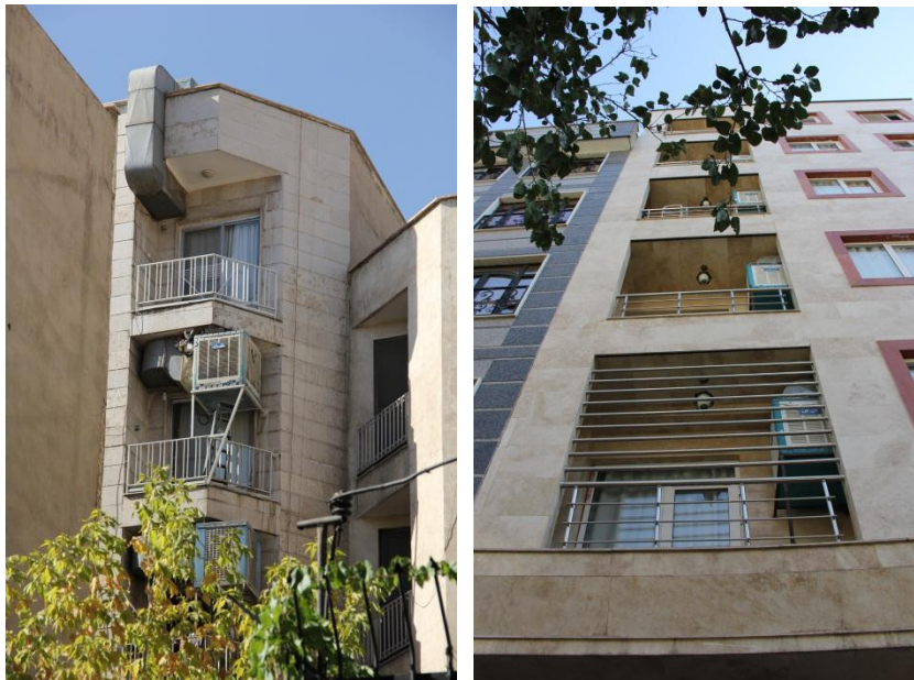
Figure 114 & 115: Misusing of Balconies. Shahrak Gharb district of Tehran. (Photo was taken by author, 2016)
