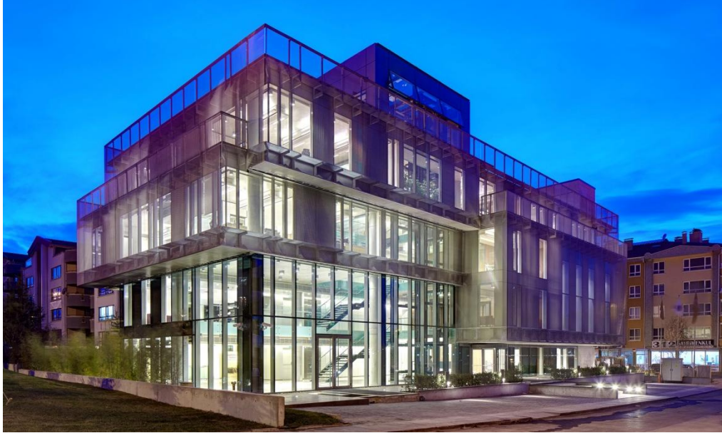
Figure 4.17 Turkish Contractor's Association Headquarters Source: Ibid.
