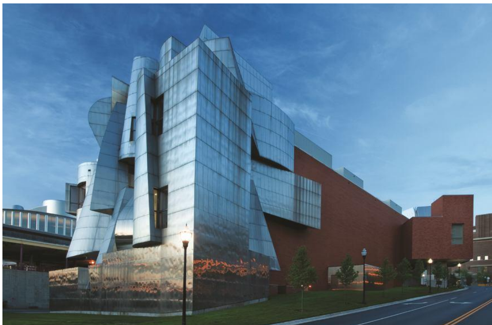
Figure 3.31 Exterior view of the Weisman Art Museum in Minneapolis with non-structural metal cladding
