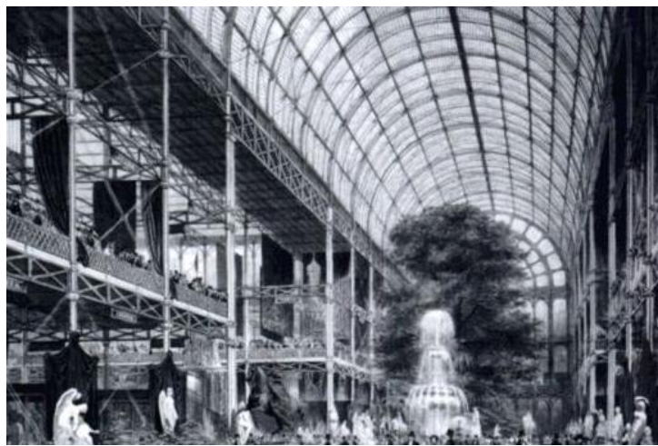
Figure 2.9 Interior of the Crystal Palace
