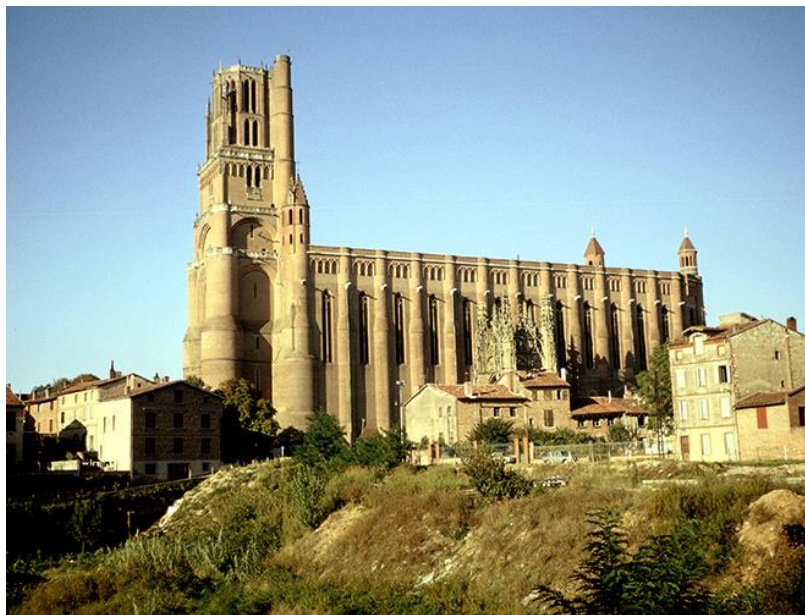
Figure 2.5 Exterior view of the Albi Cathedral
