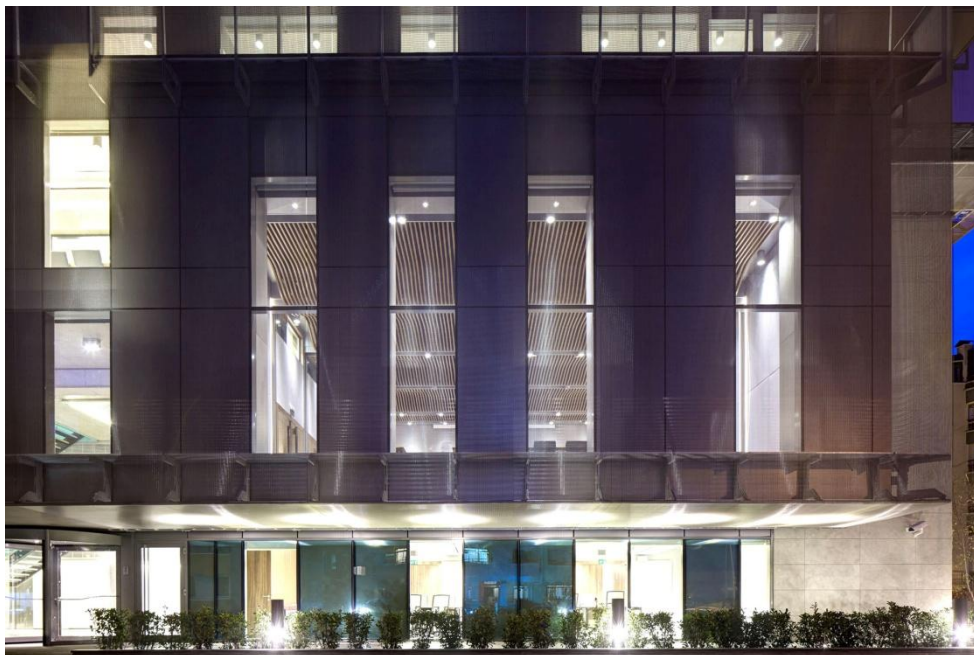
Figure 4.18 External mesh shading of the Turkish Contractor's Association Headquarters Source: Ibid.
