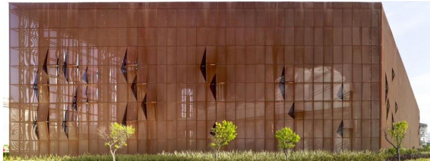
Figure 3.20 Semi-transparent, rusty facade of Raif Dinçök Yalova Cultural Center Source: Ibid.
