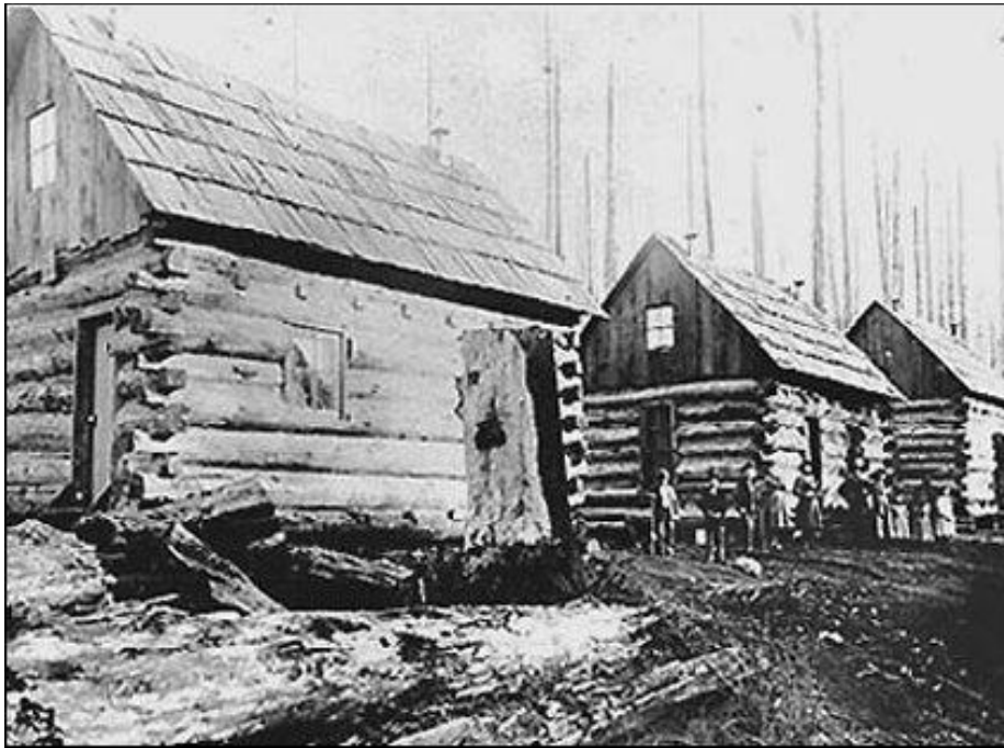
Figure 2.7 Log cabins in America as an example of the vernacular architecture
