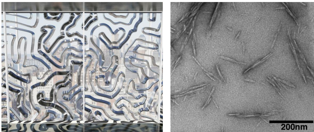
Figure 2.12 (left) Decker Yeadon's homeostatic facade system (created with smart materials) which shifts and moves according to outside air's temperature Source: Chirs Lefteri. "How Do Mysterious Memory Materials Work," ArchDaily , 2014, http://www.archdaily.com/533679/how-do-mysterious-memory-materials-work , (May 28, 2016).
