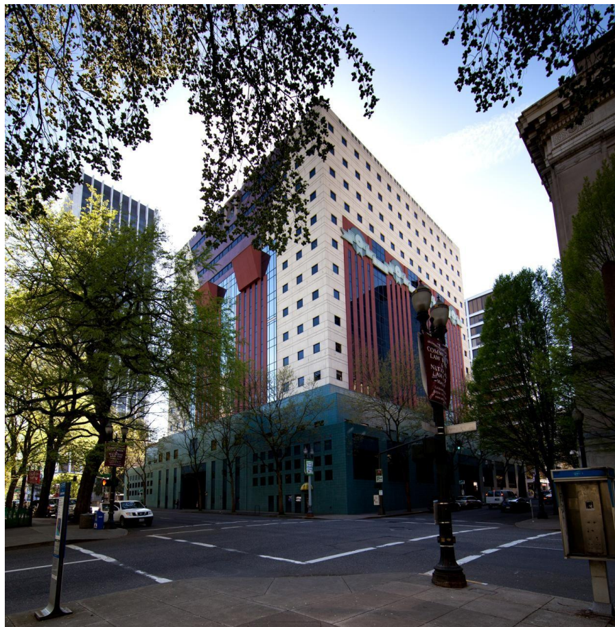
Figure 3.26 Exterior view of the Portland Building with decorations on its facade
