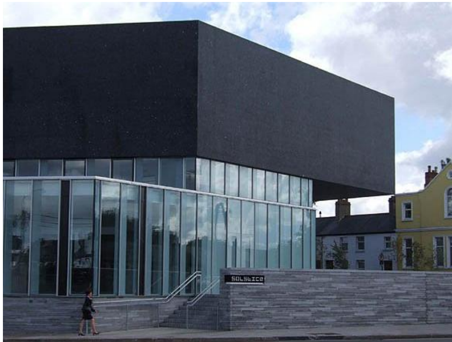
Figure 3.19 Grey-black marble mosaic slab over the civic space in uniformity with the surrounding buildings' roofs
