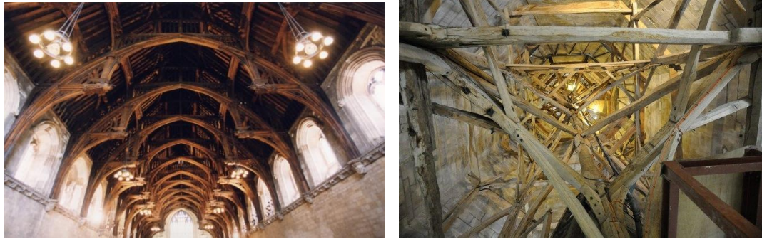
Figure 2.3 (left) Westminster Hall timber roof
