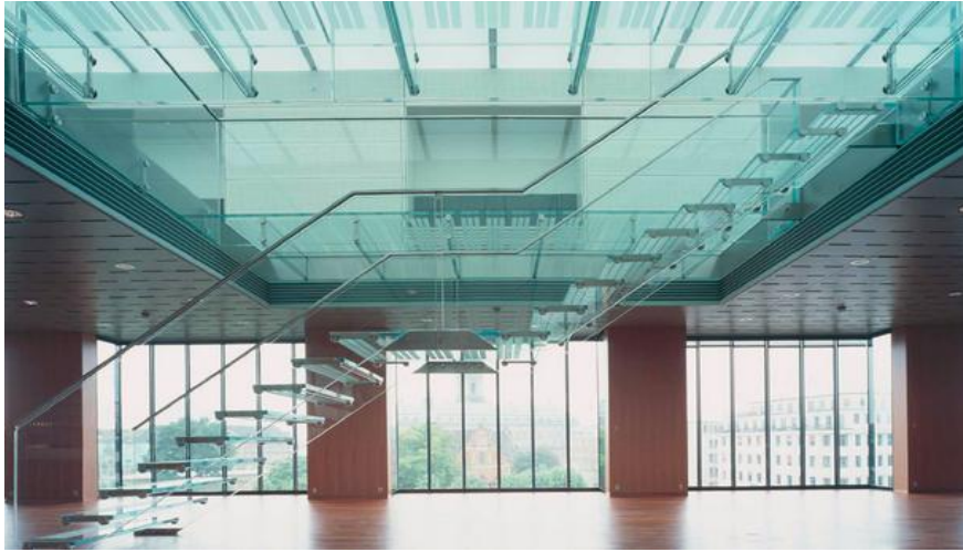
Figure 2.11 Structural glass (composite material) stairs in the Danmarks Nationalbank Source: http://www.mikkelsengroup.dk/projekt/danmarks-nationalbank-ombygning/ , (May 25, 2016).
