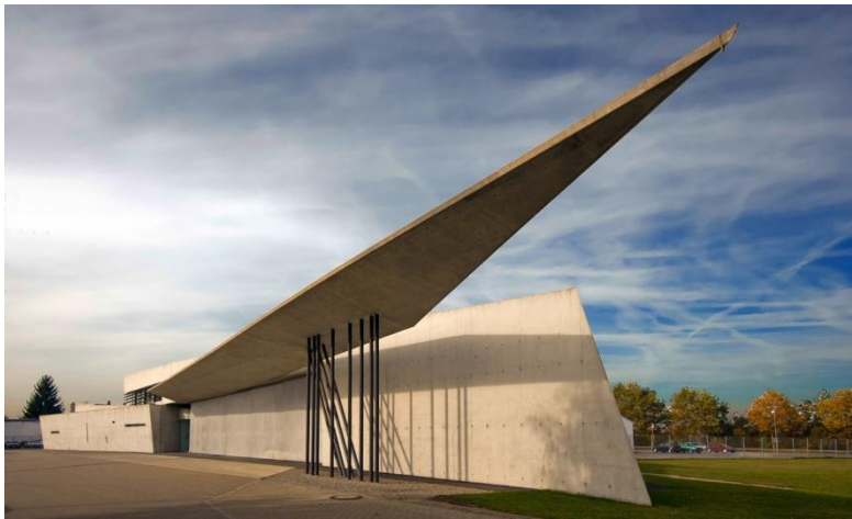
Figure 3.9 Exit door canopy of the Vitra fire station
