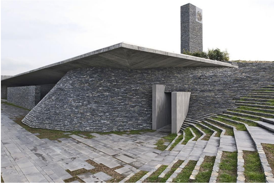
Figure 3.12 Stone roof and minaret of the Sancaklar Mosque
