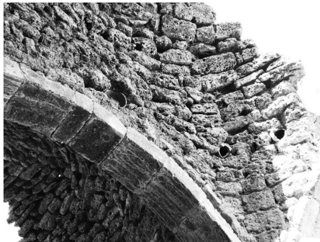
Figure 23: The pottery vessels that were inserted into the jarults, as the mouth of jar is unblocked, in Asarağaç (Kelkaya) Church (Author, 2013)
