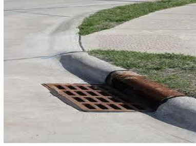
Figure 2.2 Example of Curb Inlet with grate
