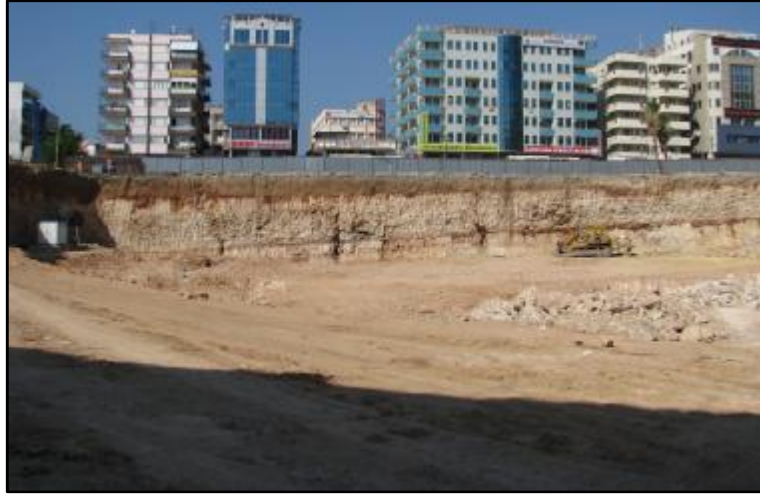
Figure 15. A view from a foundation excavation of a business center construction in the Konyaaltı district of western Antalya (August, 2008).
