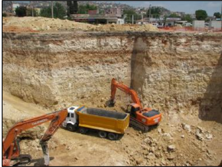
Figure 16. A view from excavations of the Antalya light railway construction (August, 2008).
