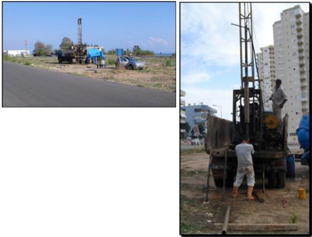
Figure 23. A view from Borehole SK-3 during drilling operations (October, 2009).
