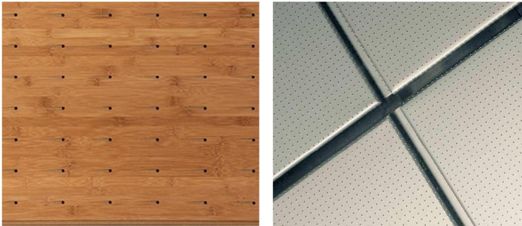
**Figure 3.4** Micro-perforated panel absorber examples
