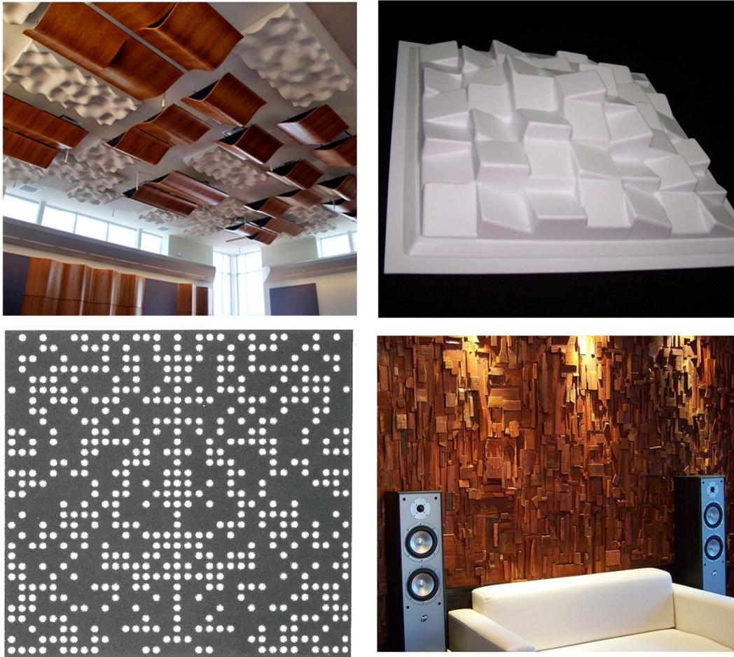
**Figure 3.5** Various acoustic diffuser examples
