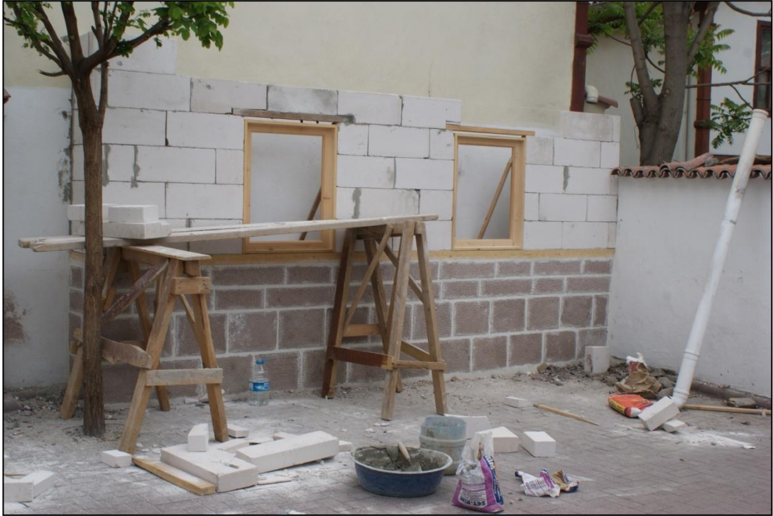
Figure 53. Construction of a Fake Façade in front of a Blind Façade
