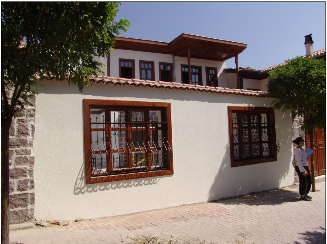
Figure 54. A Courtyard Wall Constructed as a Building Façade on Dutlu Street
