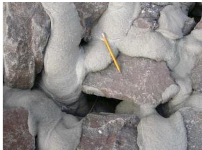
Figure 5.33 Placement of partially grouted riprap (Lagasse et al., 2007)
