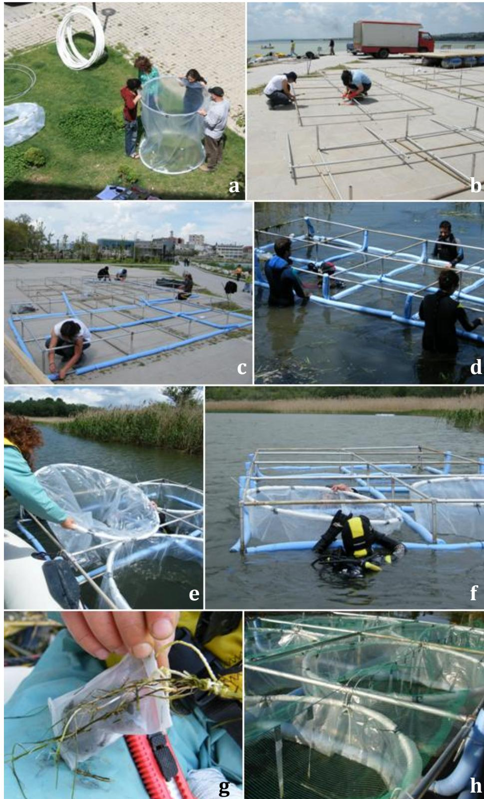
Figure 3: Steps in mesocosm construction a) setting up cylindrical enclosures, b) assembling aluminum frames, c) attaching PU foams to frames, d) placing frames on site, e-f) installing and fixing mesocosms, g) planting macrophyte shoots, h) covering mesocosms with netting
