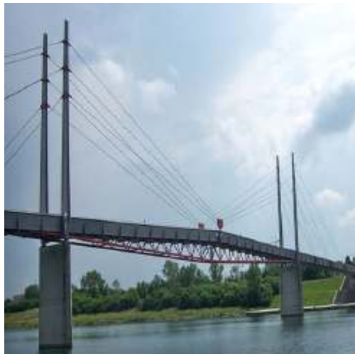
Figure 1.8 Whole view of the bridge [17]
