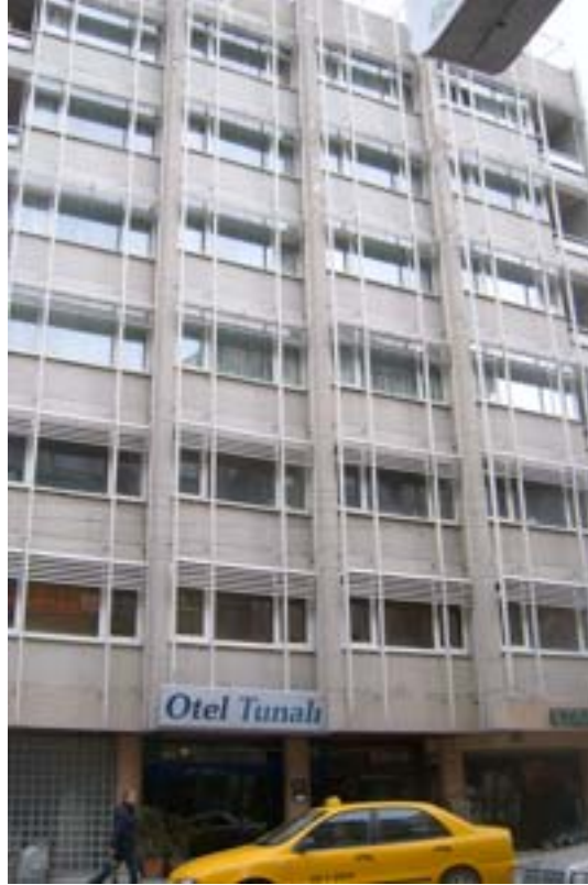
Figure 29d. Front facade, Tunalı Oteli Source: Author's archive, 2009
