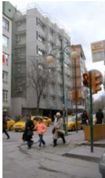
Figure 29e. Exterior view, Tunalı Oteli Source: Author's archive, 2009
