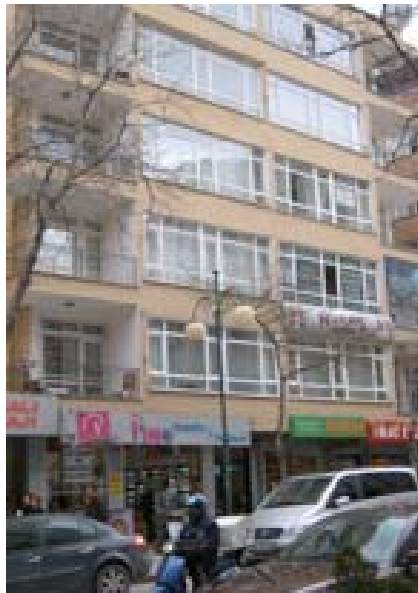
Figure 39. Tunalı Pasajı Source: Author's archive
