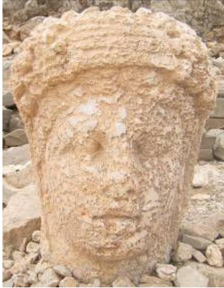
**Figure 3.5** Material losses by pitting on the head of Kommagene at the east terrace of Nemrut Dağ Monument
