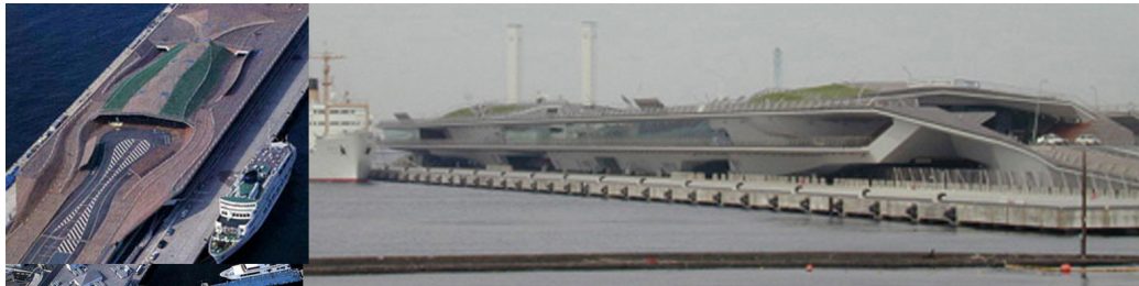
Figure 49 Yokohama International Port Terminal.
