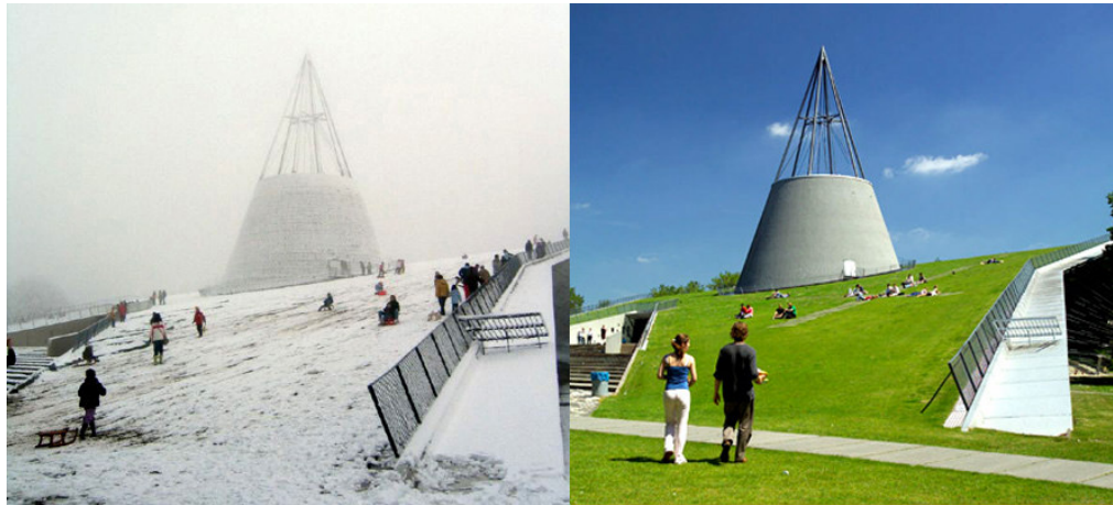
Figure 63 Images in different times from the roof of the Delft University of Technology Library. (Source: Delft University of Technology Library, Mecanoo, Retrieved January 16, 2008 from ( http://www.flickr.com/ )
