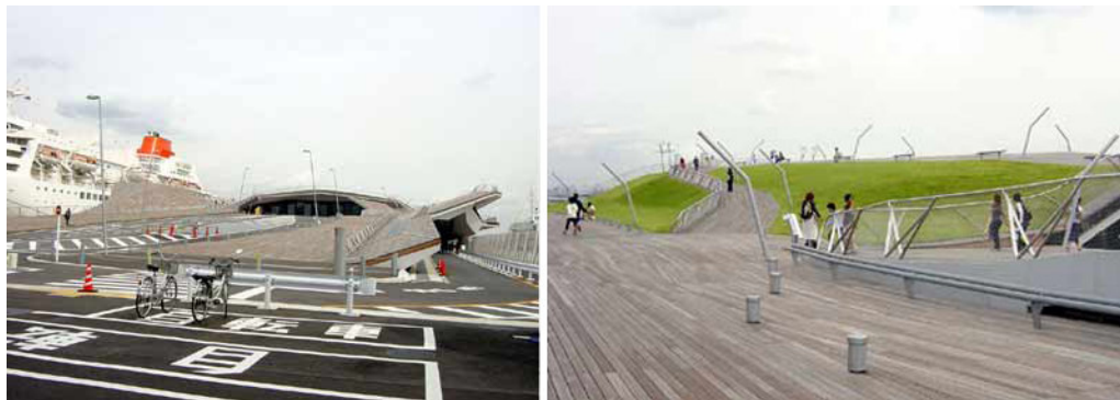
Figure 57 Yokohama International Port Terminal.
