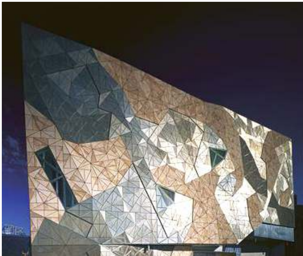
5.8. One of the built façades in sandstone, zinc and glass with the use of triangular matrix. (source: http://www.labarchitecture.com/ , accessed : November 2007. )
