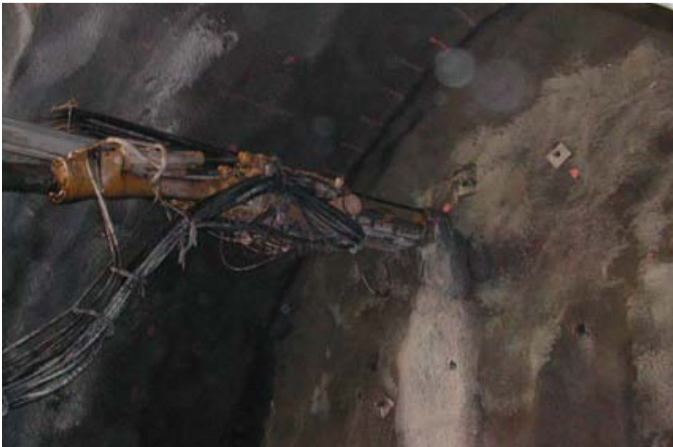
Picture A3.6 Jumbo Drill Rig Installing Face Bolts
