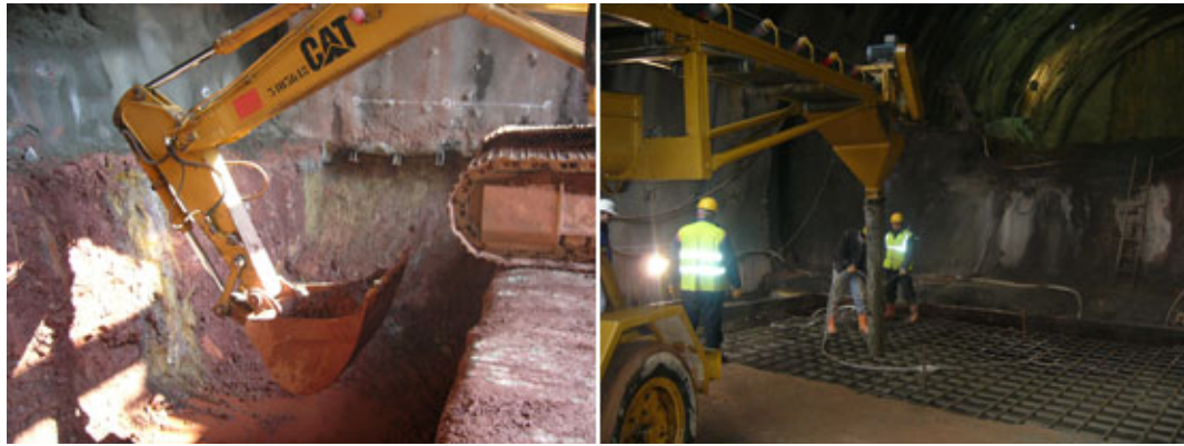
Picture A3.7 Invert Excavation
