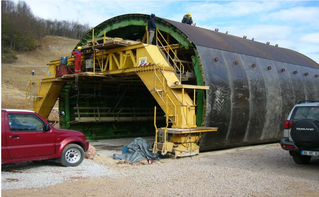
Picture A3.12 Inner Lining Form
