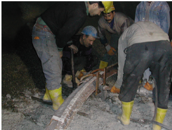
Picture A3.3 Omega TH 29 Steel Ribs
