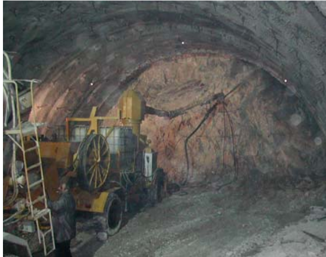
Picture A3.2 Face Sealing Application
