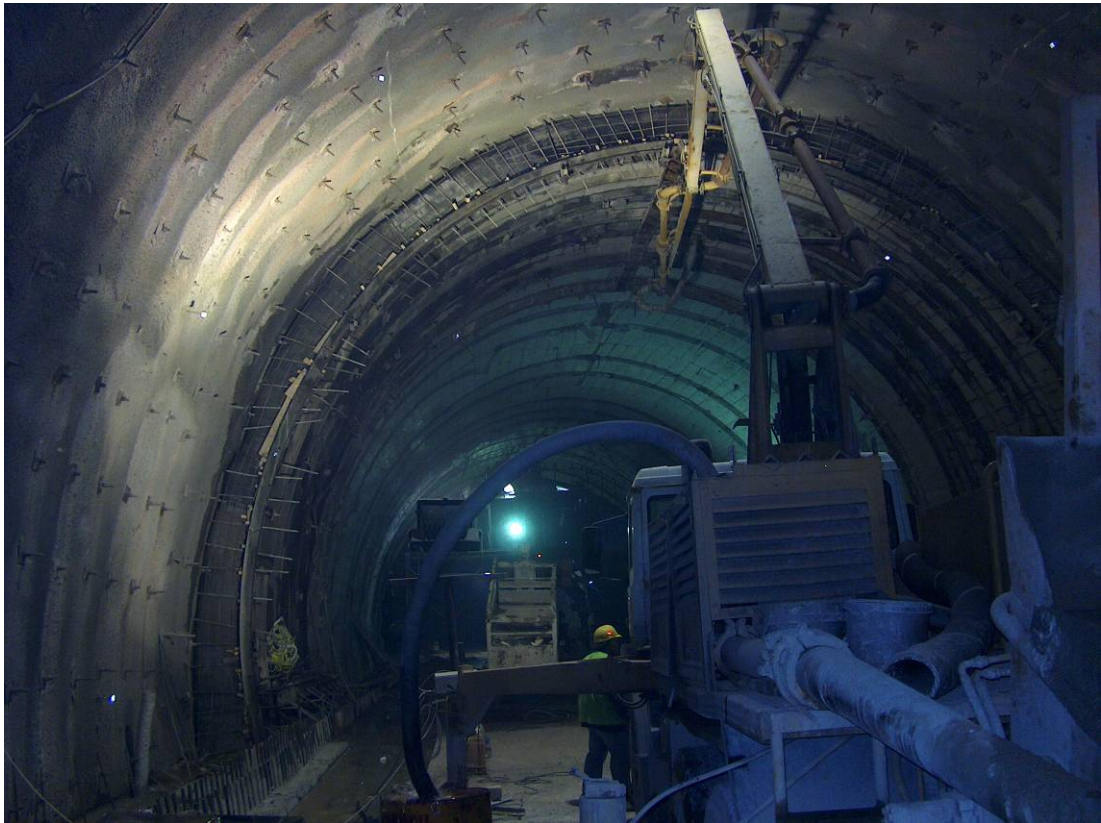
Figure A3.10 Bernold Concrete Pouring
