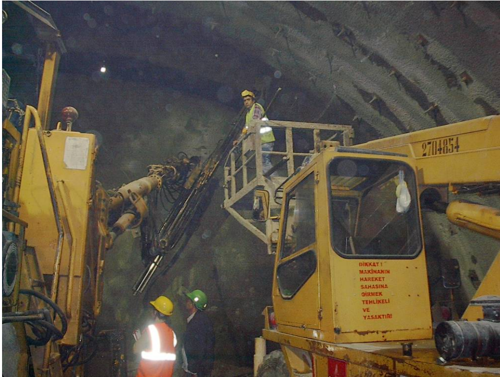
Picture A3.5 Jumbo Drill Rig Installing Round Bolts
