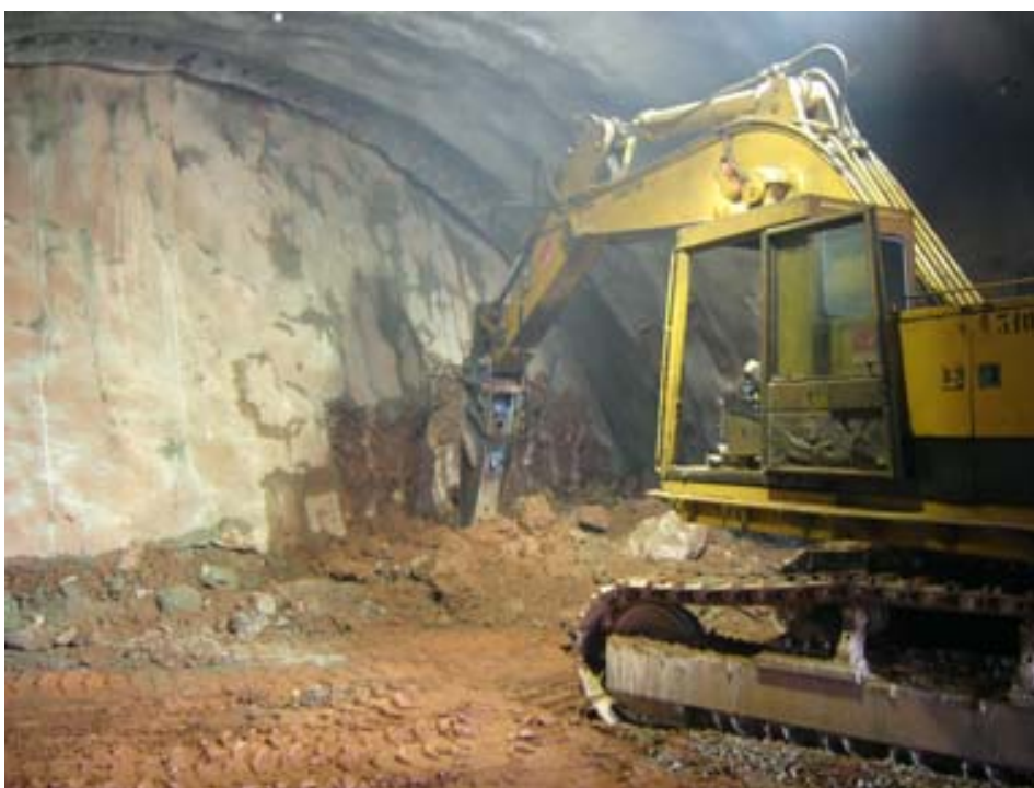
Picture A3.1 Top Heading Excavation
