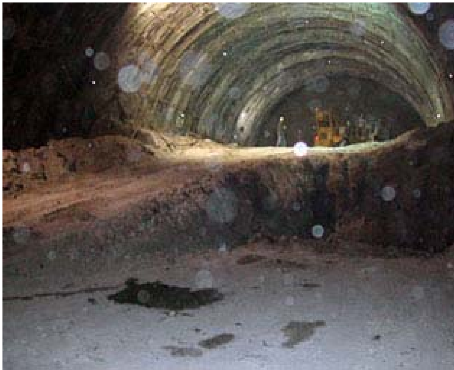
Picture A3.4 Bench Excavation
