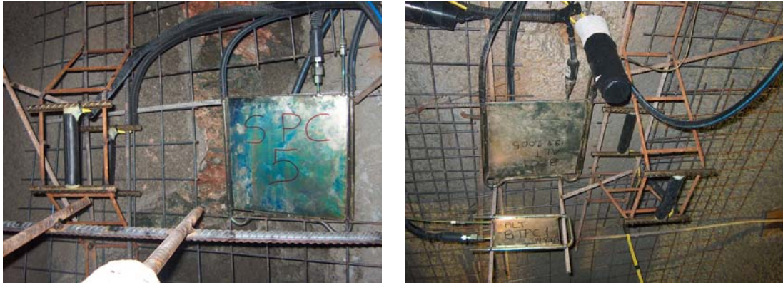
Picture A3.14 Pressure Cells and Strain Gauges
