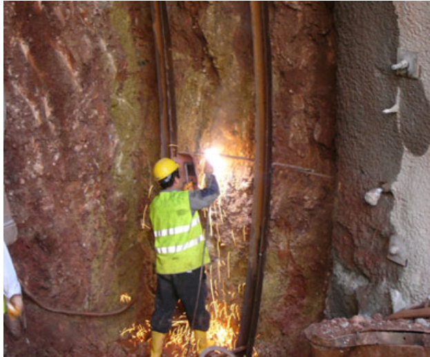
Picture A3.3 Welding of “Tie Bars”
