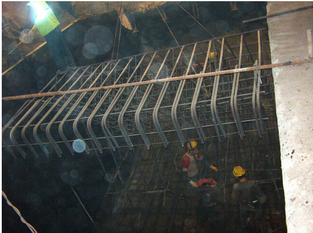
Picture A3.8 Invert Reinforcement Installation
