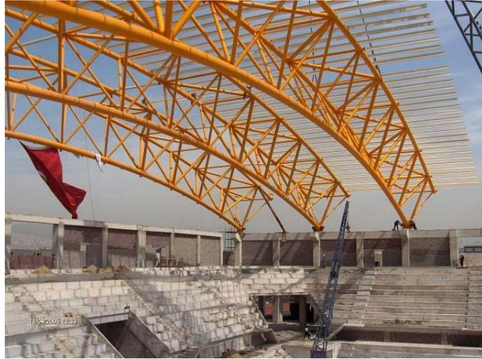
**Figure 2.3** Installations of Steel Truss Beams
