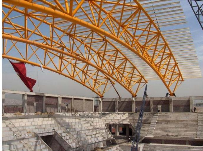
**Figure 2.3** Installations of Steel Truss Beams
