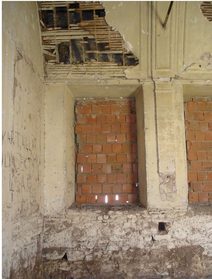
Figure-23 Window opening that closed with brick wall
