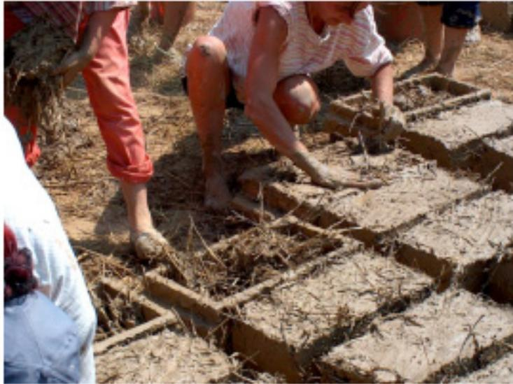
**Figure 2. 15 Production of the adobe bricks by traditional methods [16].**
