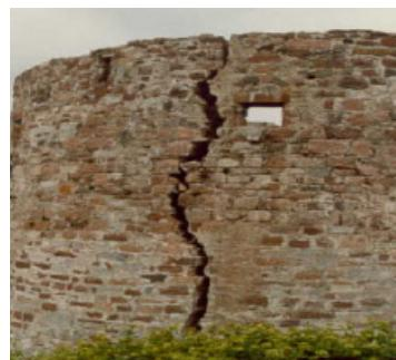
**Figure 3.13 Extended cracking along the Orta-Capu tower due to a land slide [25].**
