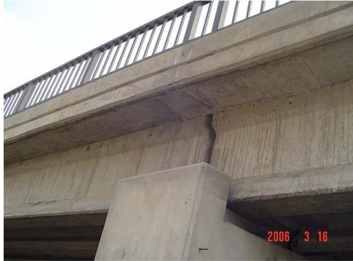
Figure 1.3: New bridge with link slab (By courtesy of Caner)
