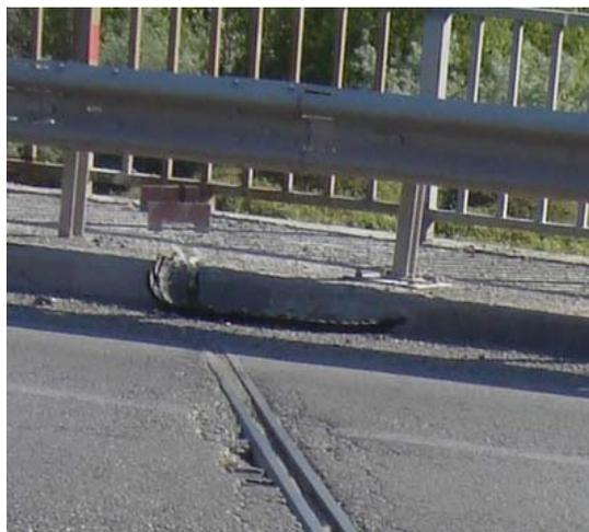
Figure 1.2: Damage in expansion joints caused by impact (By courtesy of Caner)
