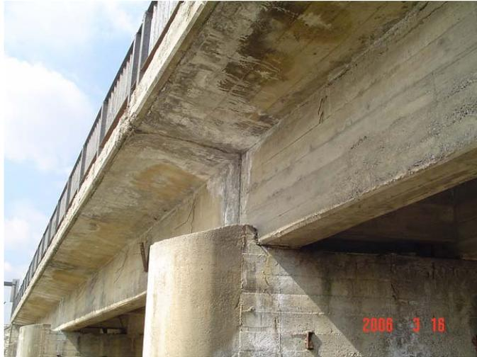
Figure 1.1: Deterioration of girder ends and cap beam at expansion joint location due to leaked water (By courtesy of Caner)
