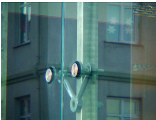
**Figure A3. Example of planar system** (Yiv Mühendislik [online]. (n.d.). from. [www.yivmuhendislik.com](http://www.yivmuhendislik.com) [Accessed at August 2006.]
