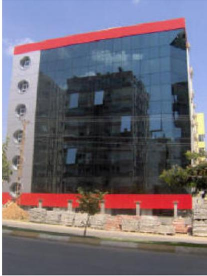
**Figure A2. Example of silicon system** (Yiv Mühendislik [online]. (n.d.). from. [www.yivmuhendislik.com](http://www.yivmuhendislik.com) [Accessed at August 2006.]
