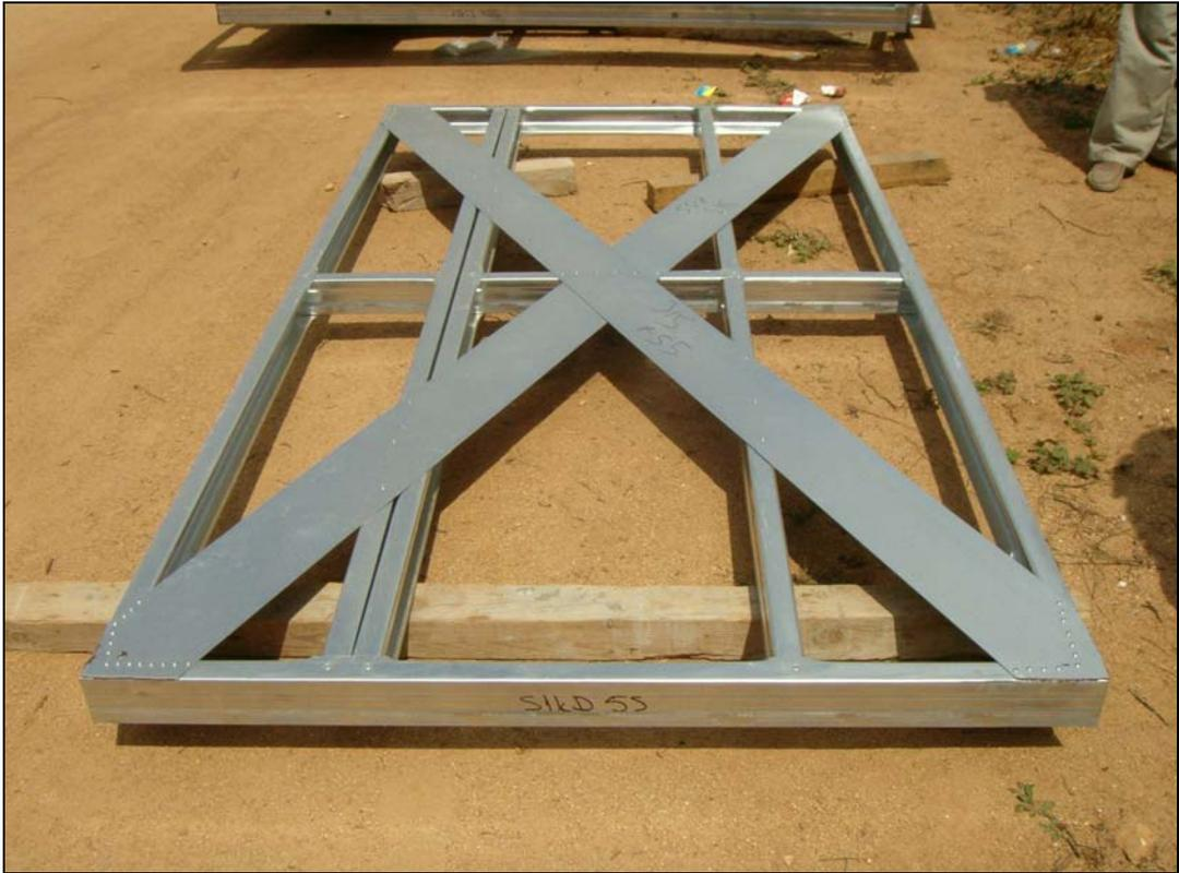
Figure 5.2 Frame with X-bracing
