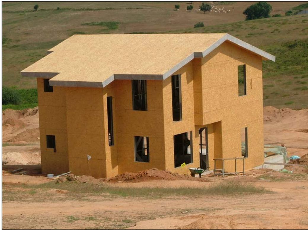
Figure 3.1 OSB Sheathed Light Gauge Steel House.
