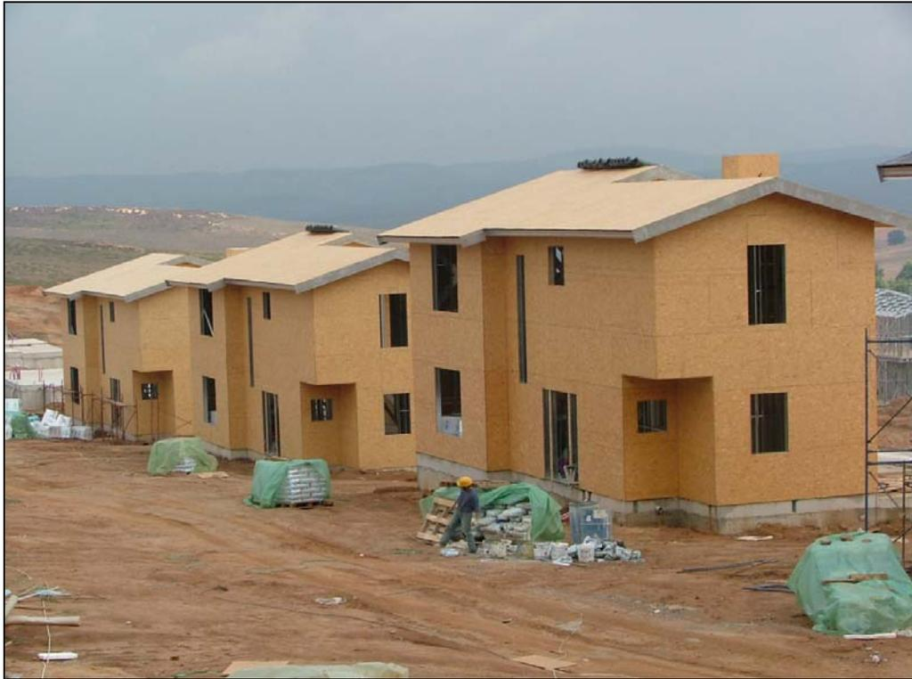
Figure 1.4 OSB Sheathed light gauge steel houses
