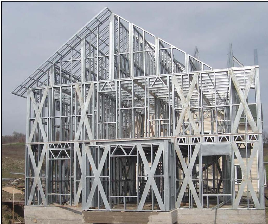
Figure 1.7 Shear Walls with X-bracing on a light gauge steel house
