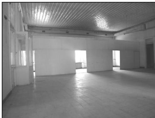
Figure 2.36 Plywood walls in space 101
