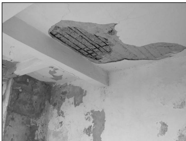
Figure 2.31 Weatherings in reinforced concrete slab
