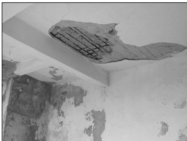
Figure 2.31 Weatherings in reinforced concrete slab
