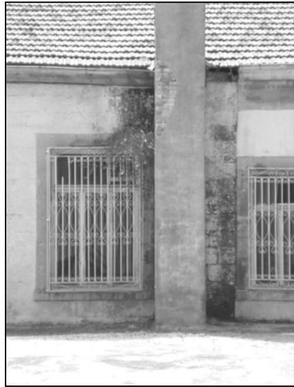
Figure 2.28 Weatherings on masonry elements Figure 2.29 Weatherings on east façade
