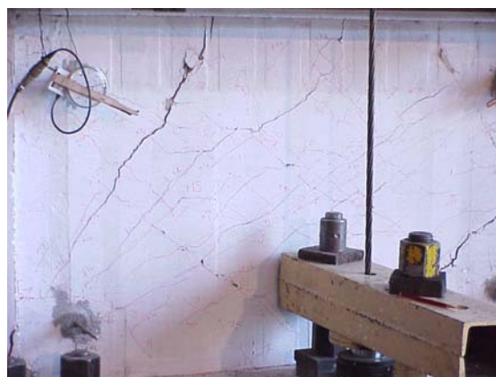
Figure 5.68 – Infill Cracking Pattern, Specimen LID4
