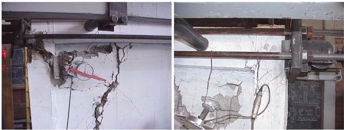
Figure 5.37 – Damage in the Beam-Column Joints after the Test, Specimen CIC4
