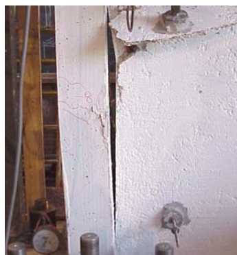
Figure 5.9 – Damage in the South Column in the Ninth Cycle, Specimen CR
