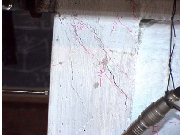
Figure 5.69 – Damage in the South Beam-Column Joint, Specimen LID4
