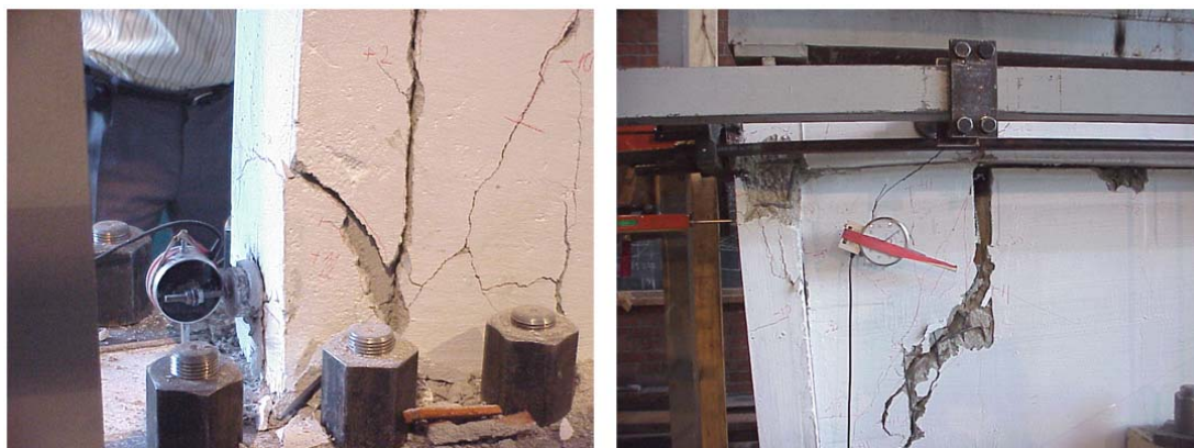
Figure 5.62 – Column Base Crack (left) and Joint Cracks (right), Specimen LIC4
