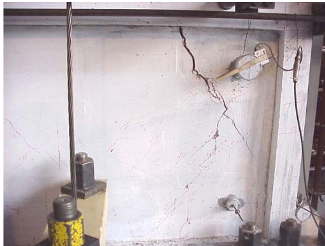
Figure 5.35 – Infill Cracks in the Seventeenth Cycle, Specimen CIC4
