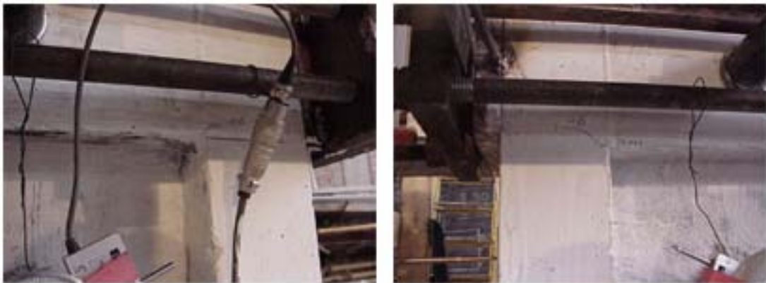
Figure 5.25 – Joint Cracks in the Sixth Cycle, Specimen CIB4
