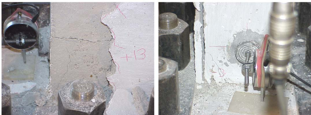
Figure 5.71 – Cracking at the Column Base and Lap-Splice Region, Specimen LID4
