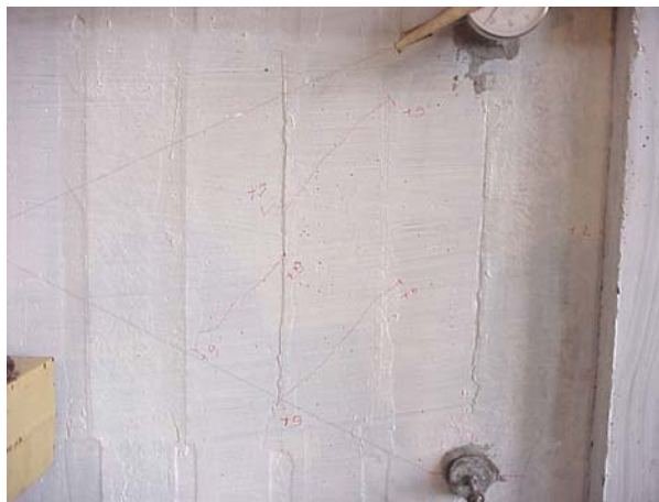
Figure 5.42 – Panel Cracks in the Ninth Cycle, Specimen CID4
