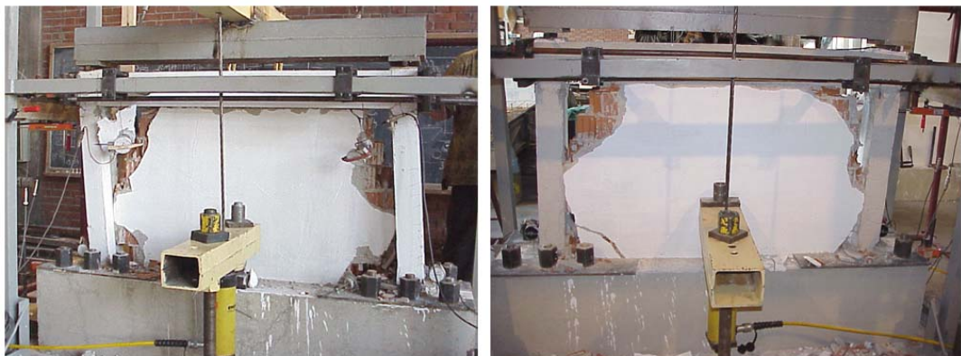
Figure 5.54 – General View of Specimen LR after the Test
