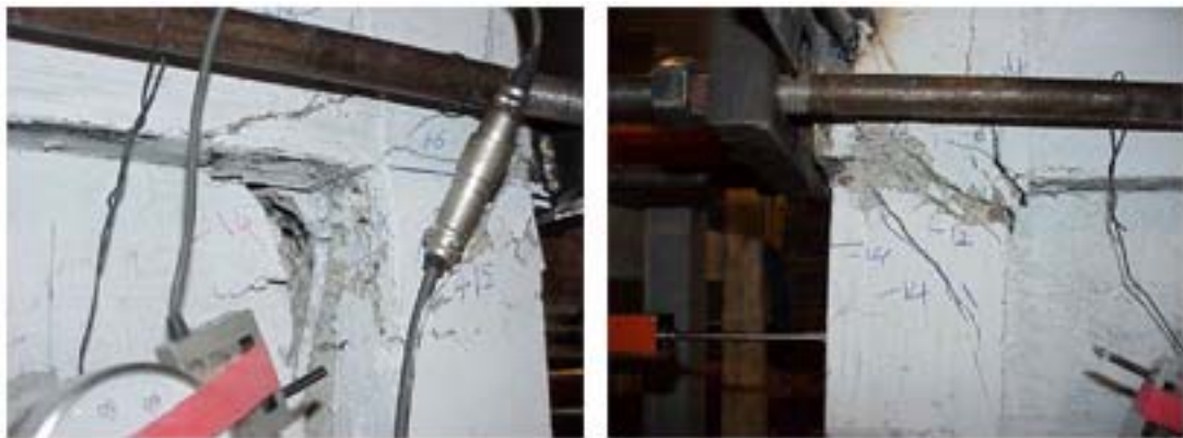
Figure 5.27 – Damage at the Joints, Specimen CIB4
