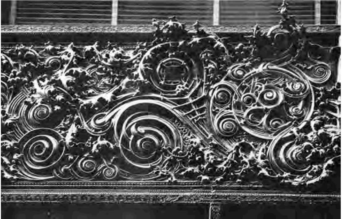
Figure 4.81. Detail, Cast iron ornamentation of the base, Schlesinger & Mayer Store (Szarkowski, 1960, p. 150)
