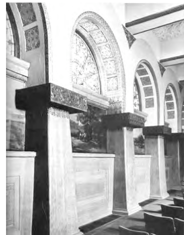
Figure 4.20. Prismatic column capitals the Auditorium Banquet Hall (Connely, 1960, p. 173)
