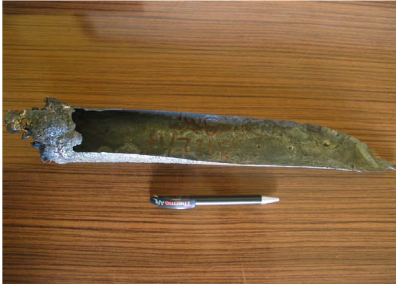
Figure 4.1 Steel sample taken from clogged nozzle.
