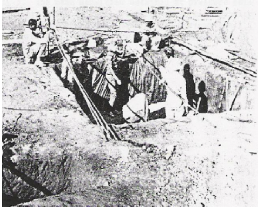
Figure 2.28 Total Pressure Cell Installation (Robertson and Wagener, 1975)
