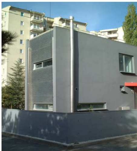
Figure16. The orientation of aluminum façade sheathing between walls in A.K. House. (Photograph by the author)
