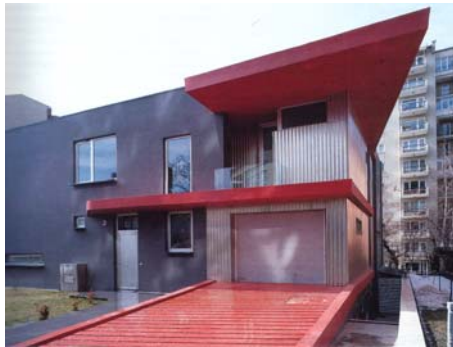
Figure15. The orientation of façade coverings between slabs in A.K. House. (Photograph by Cemal Emden in XXI , Vol.11, p. 44.)
