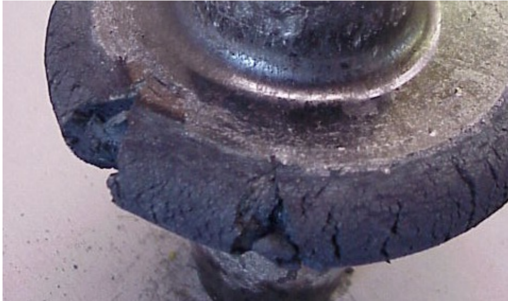
Figure 5.15 Severe cracks in the flange
