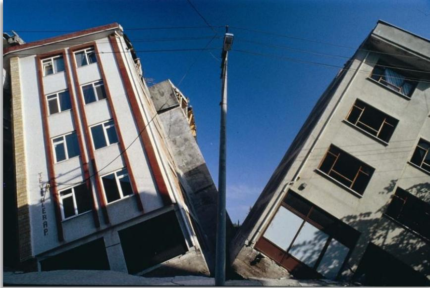
Picture 5.2 Damages in High-Rise Structures of Çark Street, Central Adapazarı (SMM, Archive)
