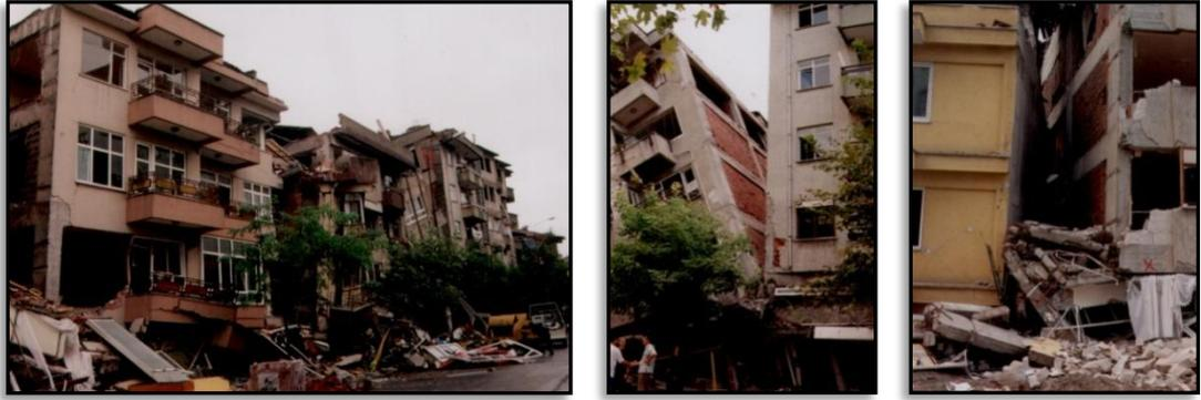
Picture 5.8 Damages in Attached Structures with Different Floor Heights
