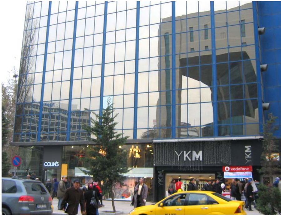
Figure 3.6. YKM Store Building, Kızılay, Ankara Source: Personal Archive.
