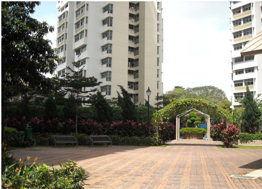
Figure 2.8. Forfar Heights, Queenstown, Singapore. (The last one among the spatial configurations which are shown above) Source: Personal Achieve.
