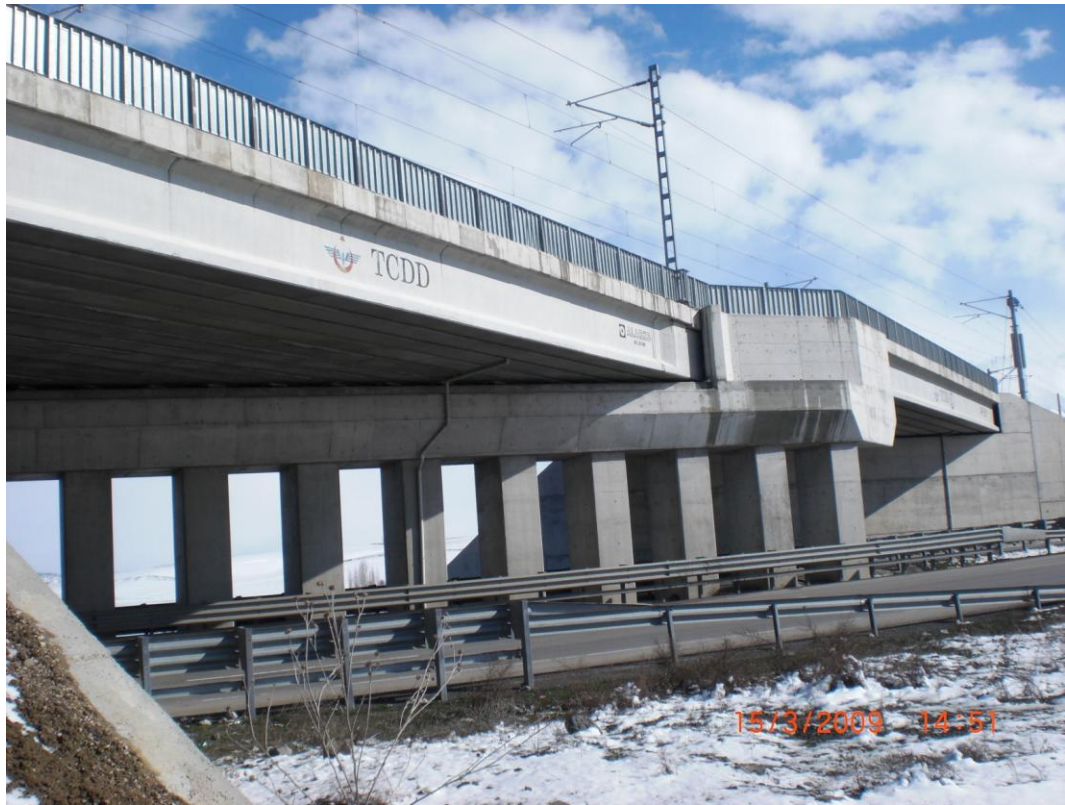
Figure 4.4 General View of Precast Concrete I-Girder High Speed Train Bridge
