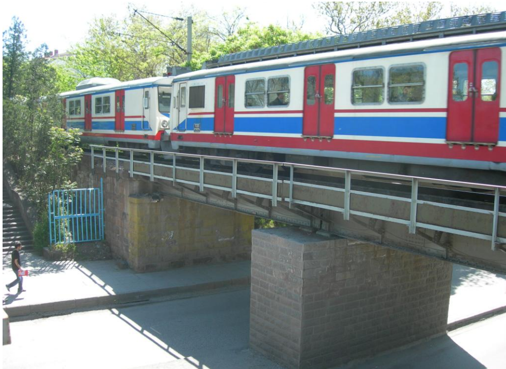
Figure 4.2 General View of Steel I-Girder Suburban Railway Bridge
