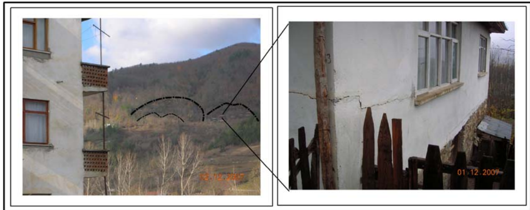
Figure 3.73. Konuklu village showing first degree of risk where the terrain show a clear movement with some indicators as house cracks
