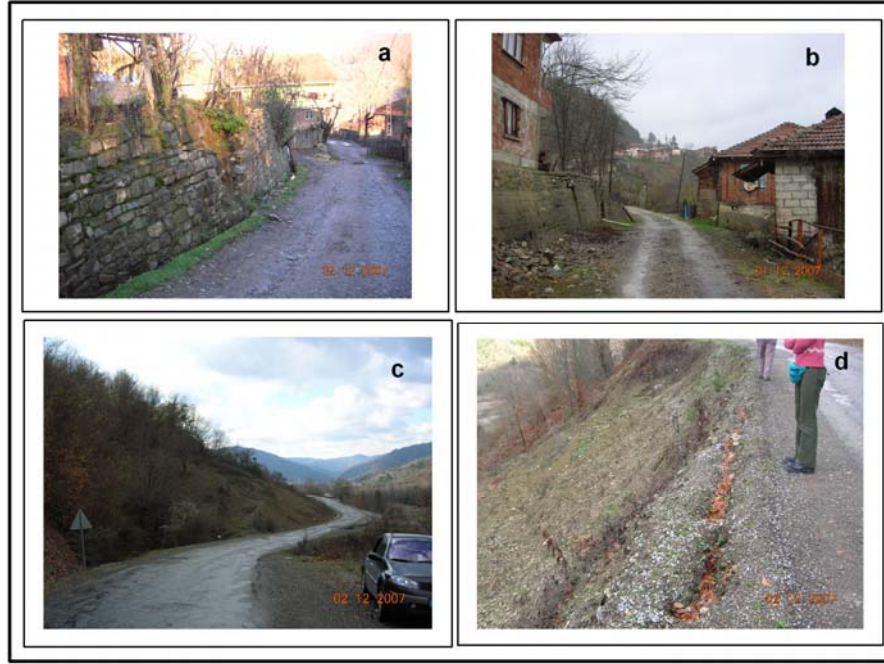
Figure 3.3. The damages observed at the road embankments and roads
