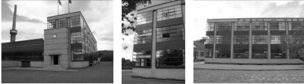
**Figure 2.17.** Fagus Shoe-last Factory: It is the first building in Europe that entirely adopted the reinforced concrete structure and glass curtain-wall. Thus it possesses great significance in architectural and construction history (Wang, Jiang, 2007)
